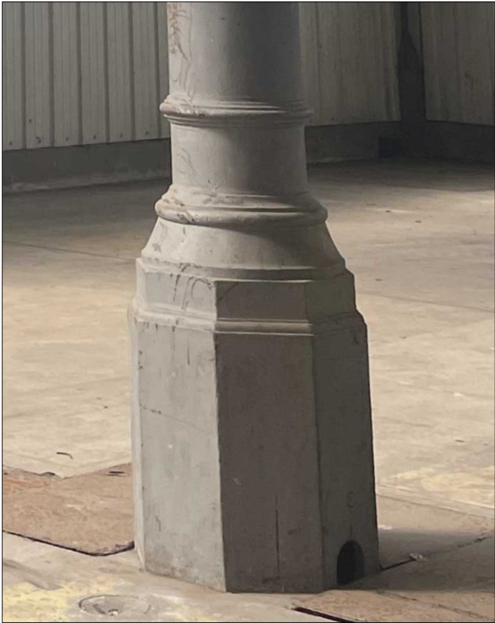
EXISTING PHOTO: COLUMN TYPE B
