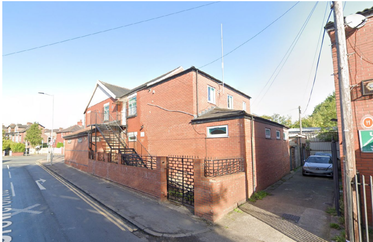
Rear/ Side of Building with rear access
