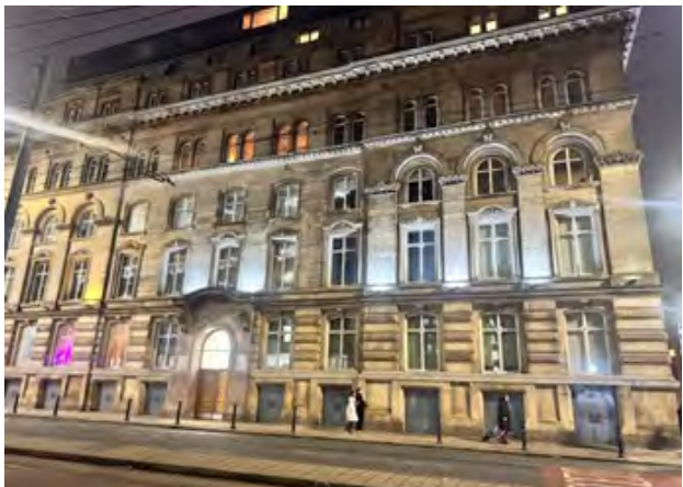
The Grand Hotel (Aytoun Street) Grade 2 listed. Facade lighting - spots fixed to historic fabric with visible cables.
