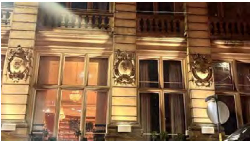
43 Spring Gardens Grade 2 listed. Facade lighting - downlights fixed to front pilasters & uplights fixed low level to historic fabric.
