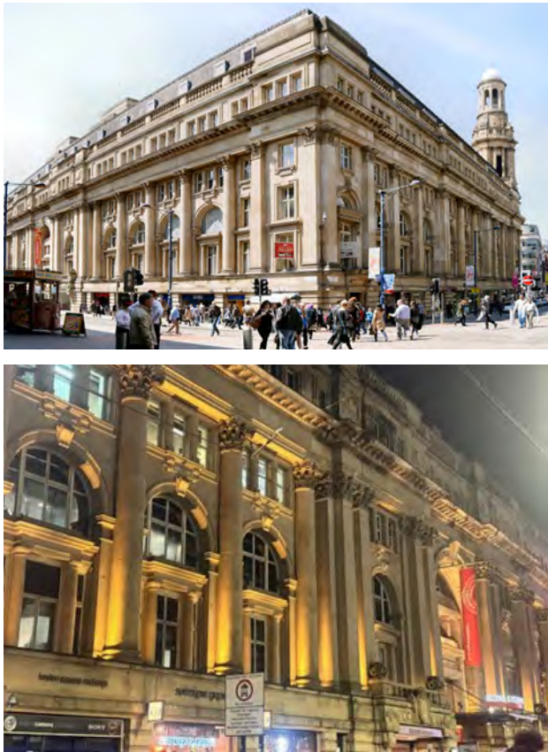
Royal Exchange Grade 2 listed. Facade lighting - uplighters fixed to historic fabric.
