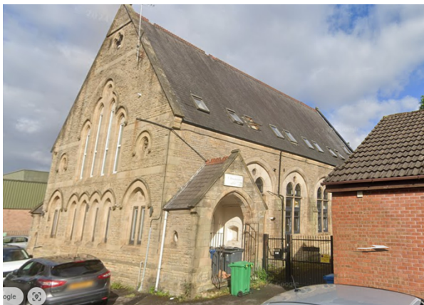
Former Chapel western elevation
