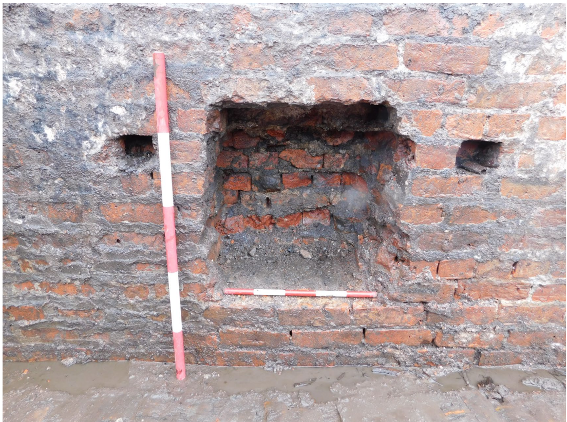
Plate 32: Cut-outs within wall [241] scales: 1m, 0.50m
