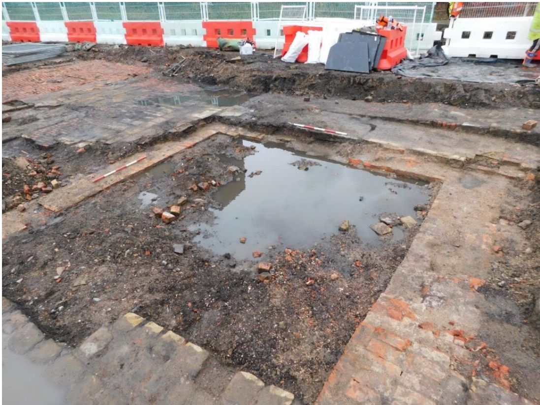
Plate 25: The walls of the extended engine house [2054] facing east, 1m and 1m scale
