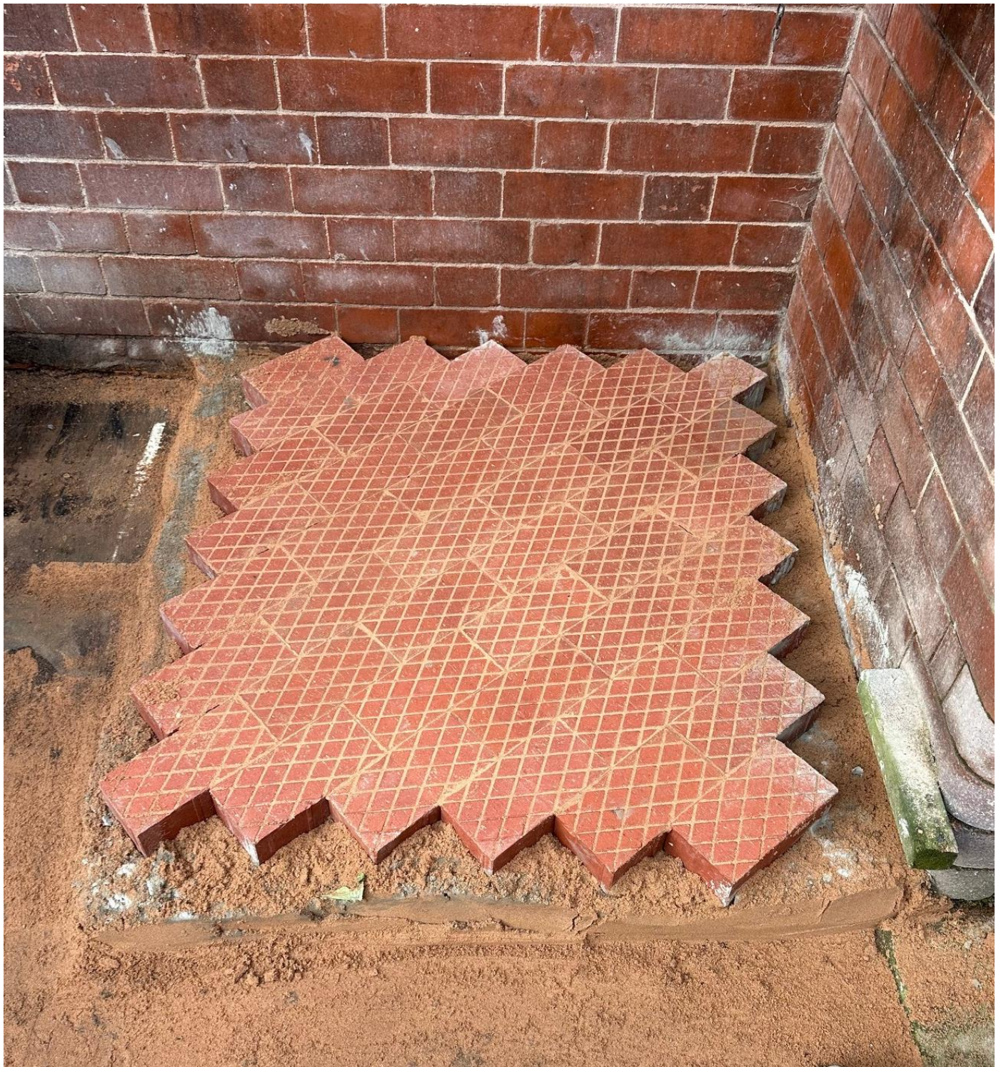
Figure 10 – Benchmark sample of new courtyard paving
