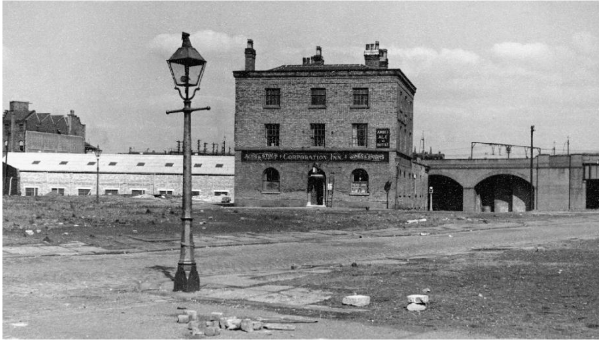
Figure 13: Corporation Inn, 1956, situated on the corner of Tipping Street and former New York Street. The photograph illustrates the post-war clearance of the built form within the Site, and the viaduct connecting to Mayfield Station to the north-west. Source: Greater Manchester Lives, ref. m49443.
