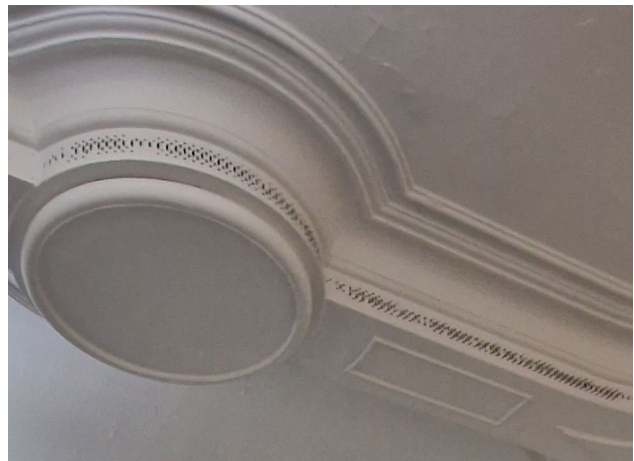
Figure 1 Photograph of the existing metal grilles to the downstand beams
