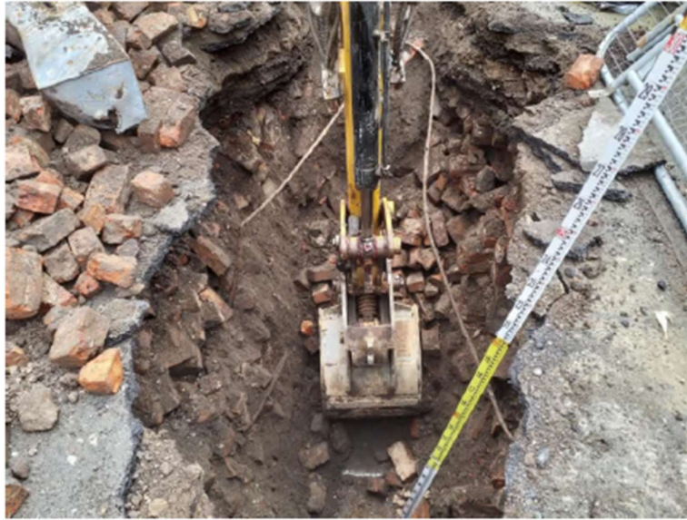
TP02 – Concrete Slab
