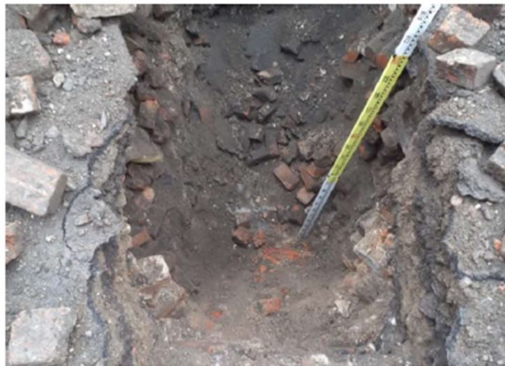
TP03 – Concrete Slab
