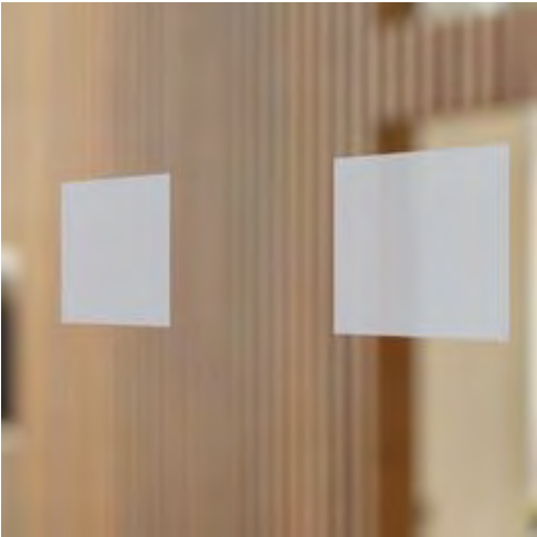
Square 50x50mm manifestation applied to glazing
