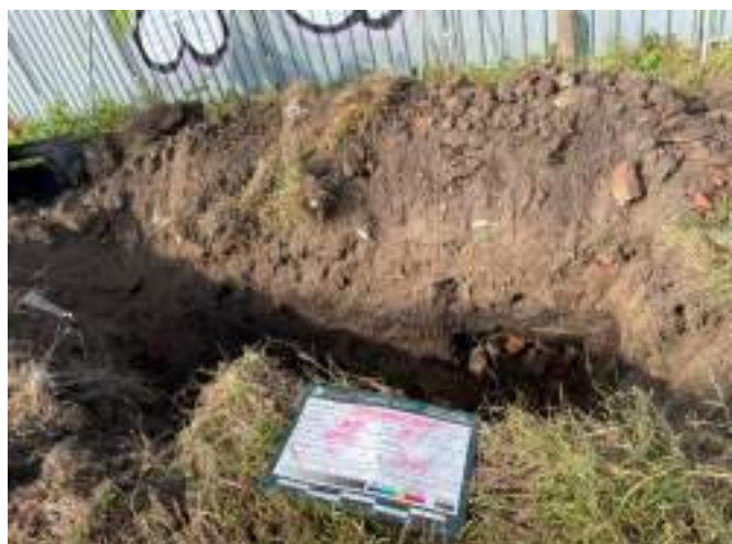
Soak Away 1: View of excavation
