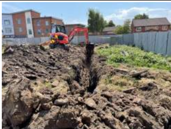
Trench 5A: View of excavation
