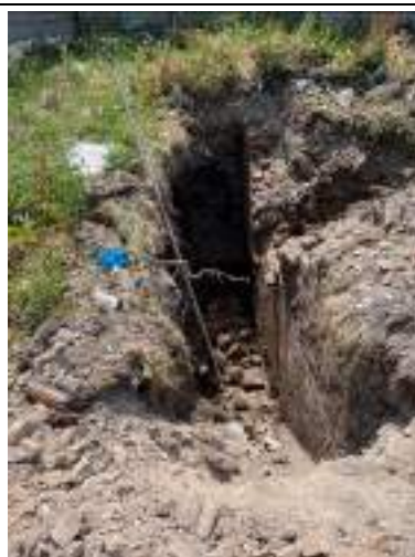
Pit C: View of excavation
