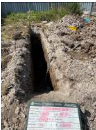
Trench 4: View of excavation
