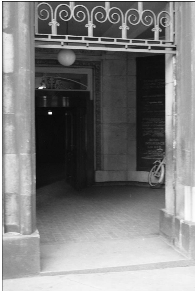
Figure 23 - Photograph dating to 1958, showing the original lobby.
