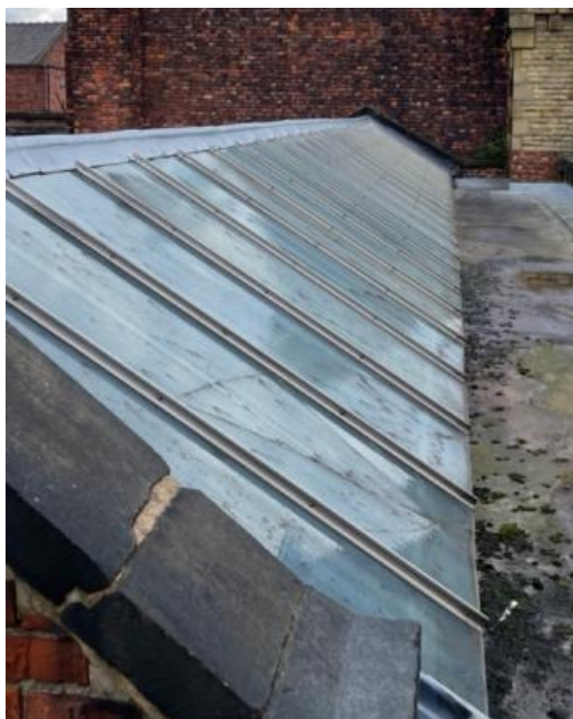
Figure 3: Existing Second-floor Roof Light
