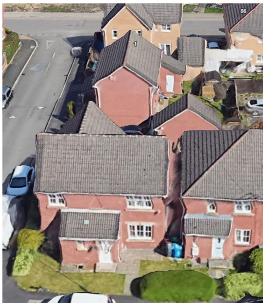
Figure 2, Existing view from no.1 Vasser Road looking onto the applicant site
