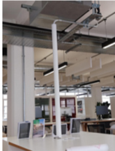
PHOTO 8 - POWER POLE EXAMPLE
