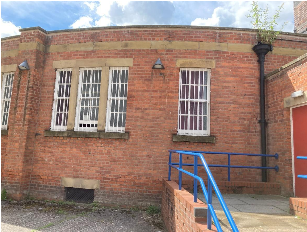
Image 01 – Ladder Access Location Nr.1
