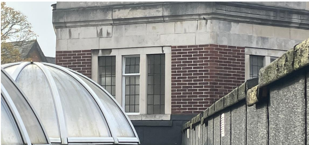
Image 03: Withington Library Existing Steel Framed Windows
