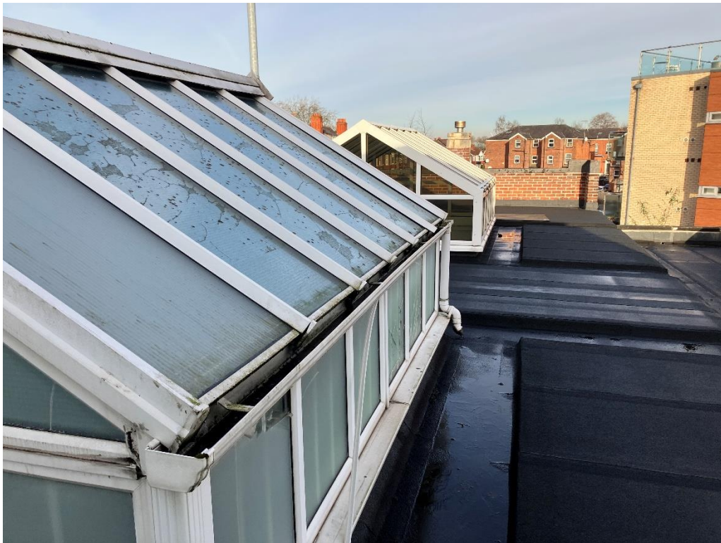
Image 03 – Roof Area to Receive ASHP Nr.1
