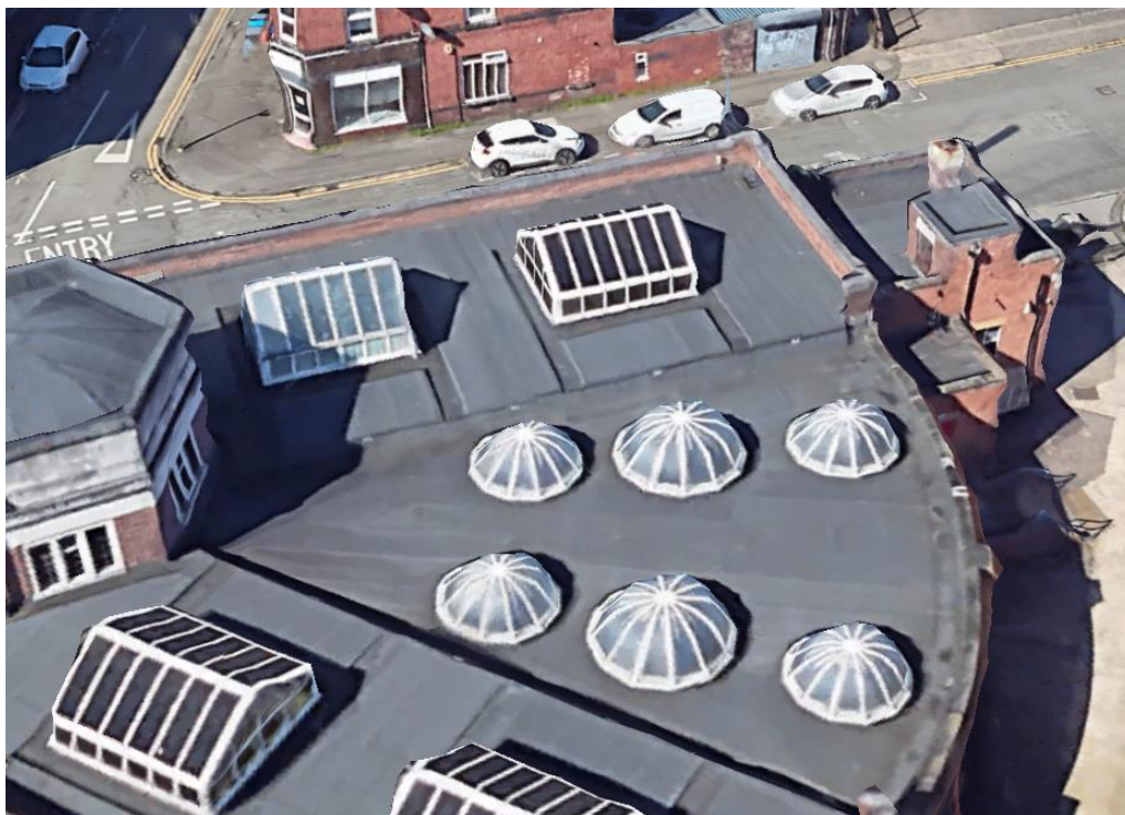
Image 05 – Roof Area to Receive ASHP Nr.3
