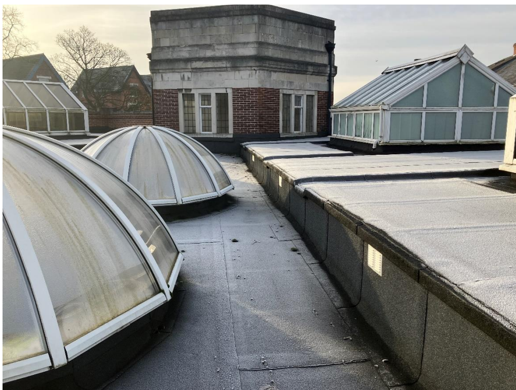
Image 04 – – Roof Area to Receive ASHP Nr.2
