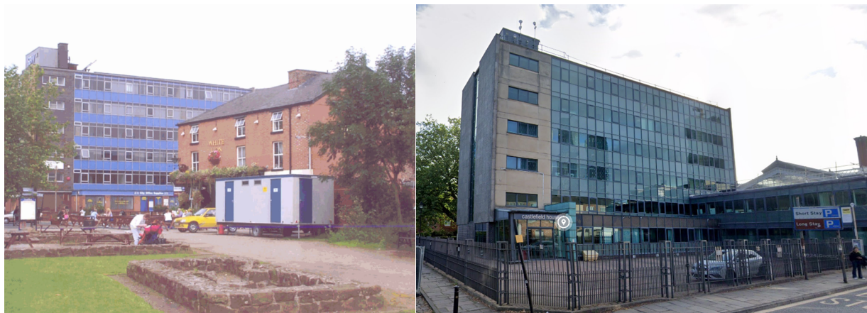
Application site as of 2003 with original façade and post refurbishment
