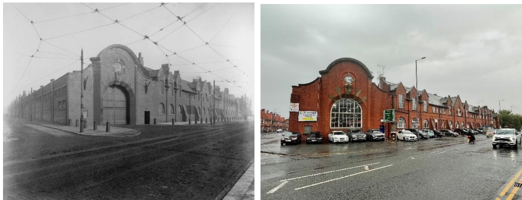
Figure 4.2: Views of the south elevation of the former tram shed (now bus depot) from the south west on Queens Road; 1902 (left) and present day (right).
