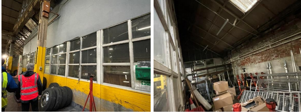
Figure 5.6: Views of the storage rooms/back of house areas within the Bus Depot
