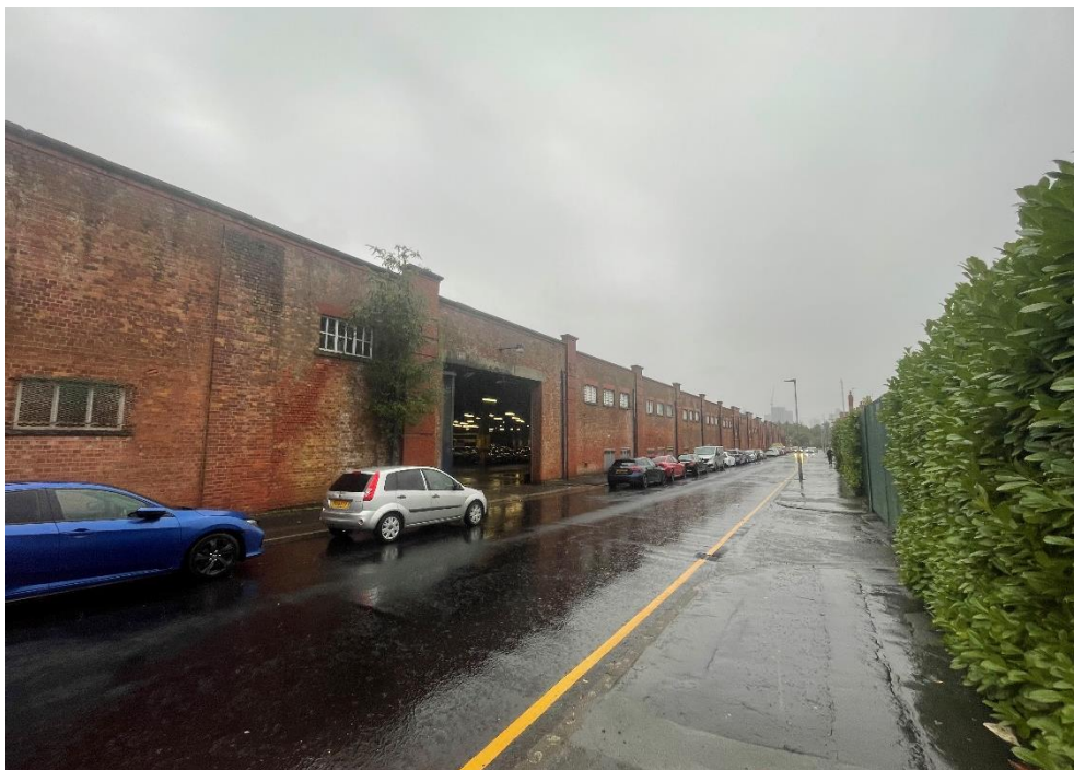
Figure 4.7: View of the west elevation of the former tram shed from the north west on Boyle Street.
