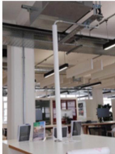
PHOTO 8 - POWER POLE EXAMPLE
