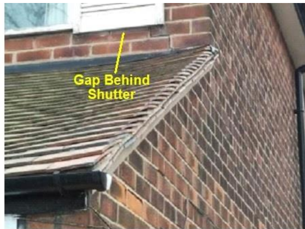
PHOTO 2 Lower Western Elevation
