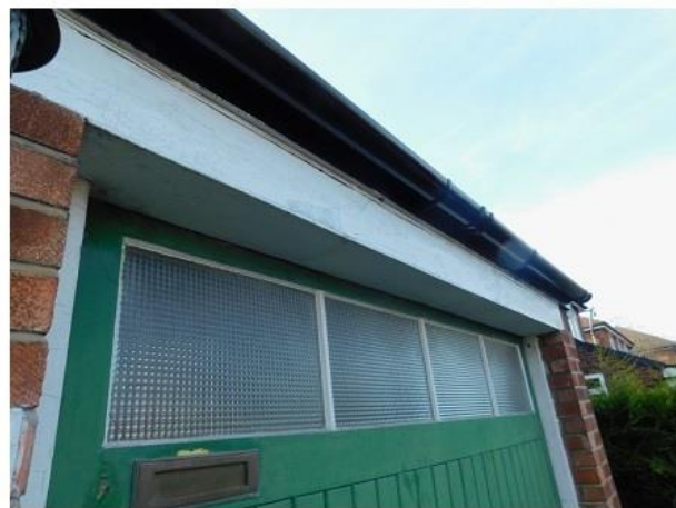
PHOTO 6 Underside of Garage Shutter Soffit
