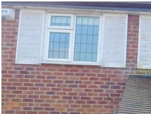
PHOTO 11 Northern View of Window Shutters
