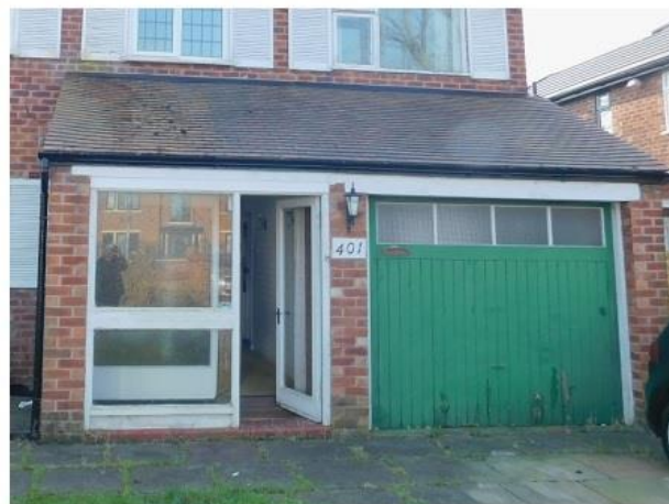
PHOTO 4 Northern Elevation of Garage and Porch
