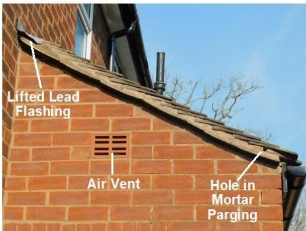
PHOTO 15 Upper Southern Elevation of WC Extension
