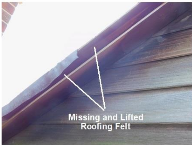
PHOTO 25 Upper North-eastern Corner of Shed
