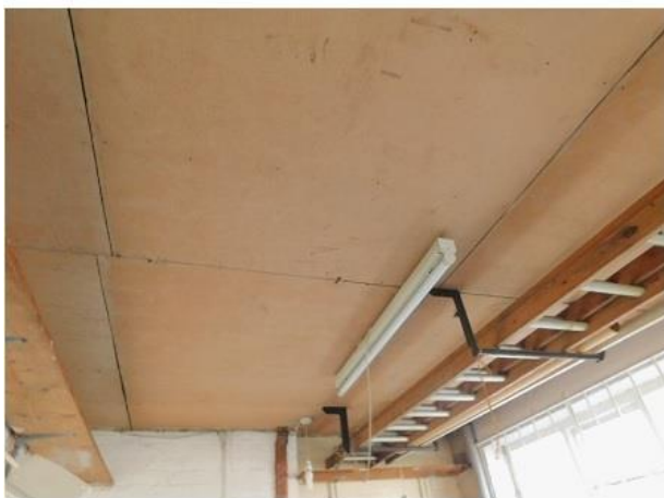
PHOTO 5 Underside of Garage Roof
