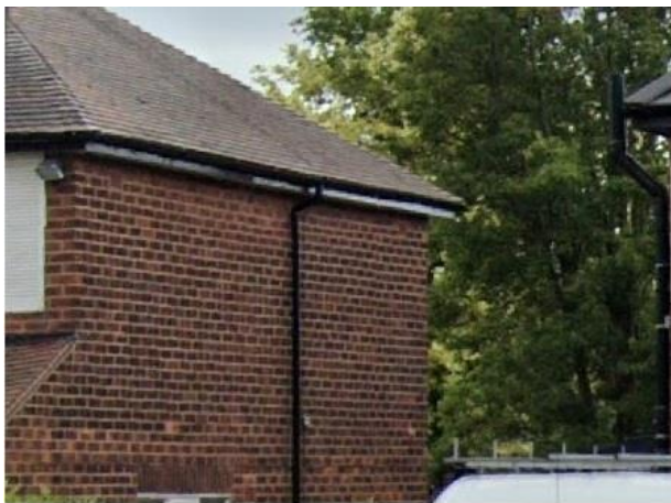
PHOTO 1 Upper Western Elevation
