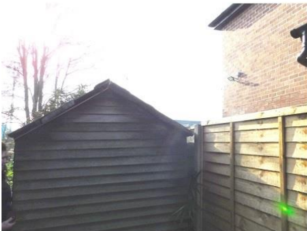
PHOTO 23 Northern Elevation of Shed
