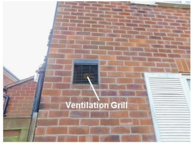
PHOTO 10 North-eastern Corner of Dwelling
