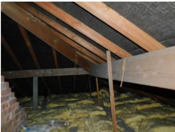
PHOTO 21 North-western Corner of Roof Void
