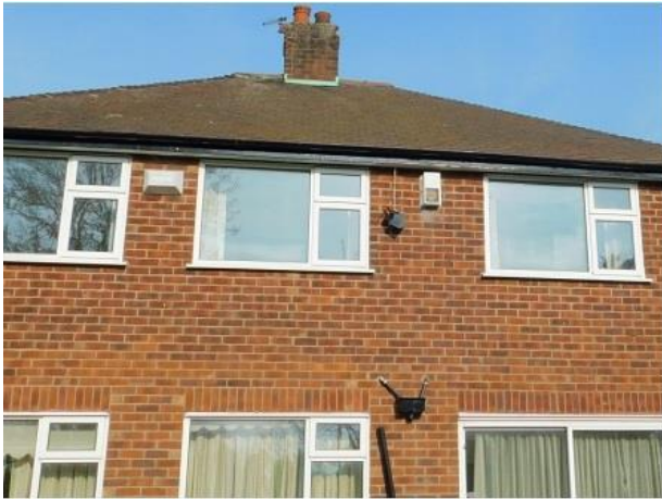
PHOTO 19 View of Southern Soffit
