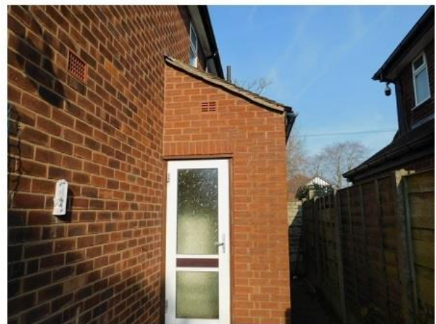
PHOTO 16 Southern Elevation of WC Exxtension
