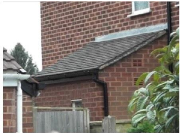
PHOTO 14 North-eastern Corner of WC Extension
