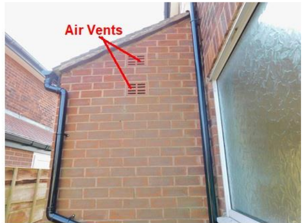
PHOTO 12 Northern Elevation of WC Extension
