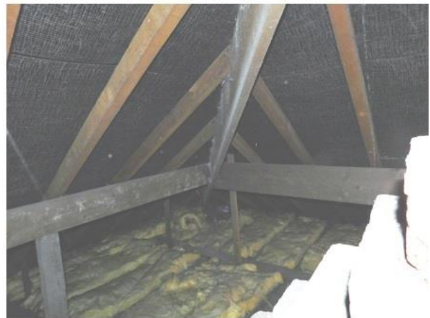
PHOTO 22 South-western Corner of Roof Void
