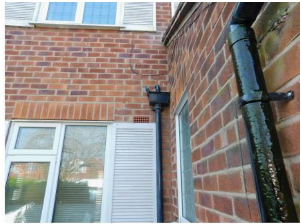
PHOTO 8 South-eastern Corner of Porch
