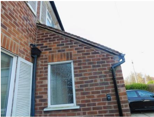
PHOTO 7 Eastern Elevation of Porch
