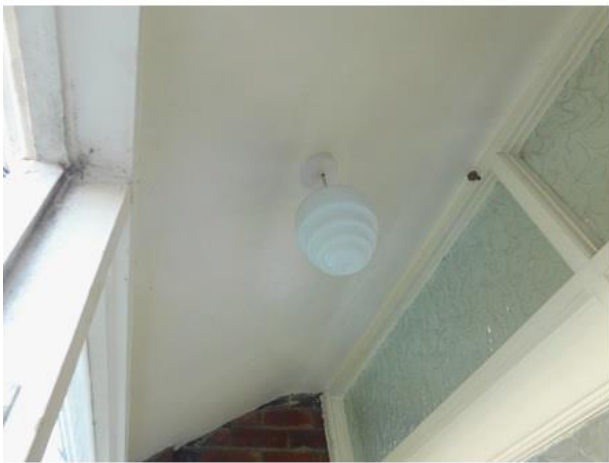
PHOTO 9 Underside Porch Ceiling
