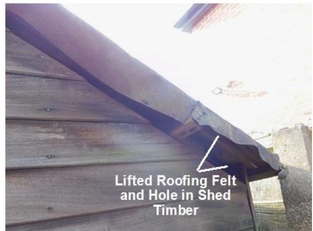
PHOTO 24 Upper North-western Corner of Shed
