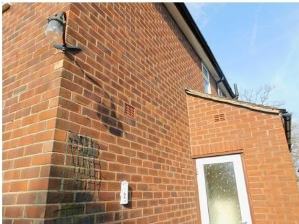
PHOTO 17 Upper South-eastern Elevation
