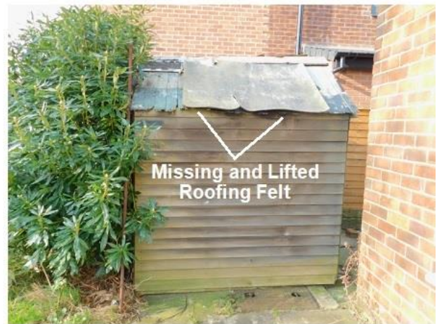
PHOTO 26 Eastern Elevation of Shed
