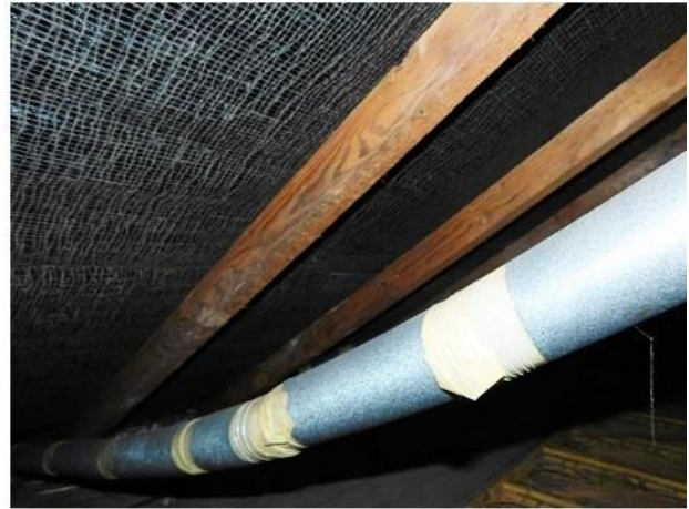
PHOTO 20 Underside of Eastern Roof
