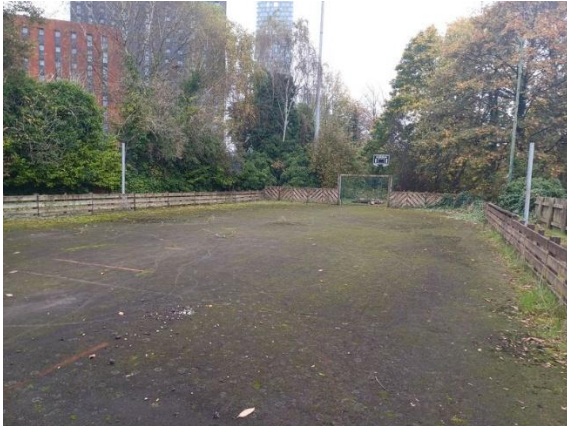
Plate 8.1: Artificial Playing Pitch with Some Signs of Wear and Encroaching Vegetation
