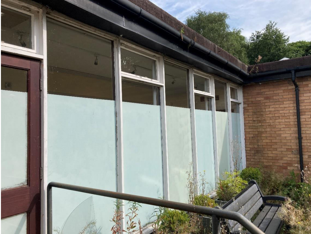
Image 05: Office & Yard Original External Windows and Doors
