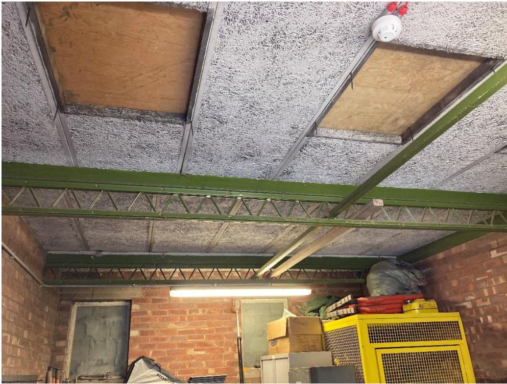
Image 02: Office & Yard Woodwool Slab Roof Deck
