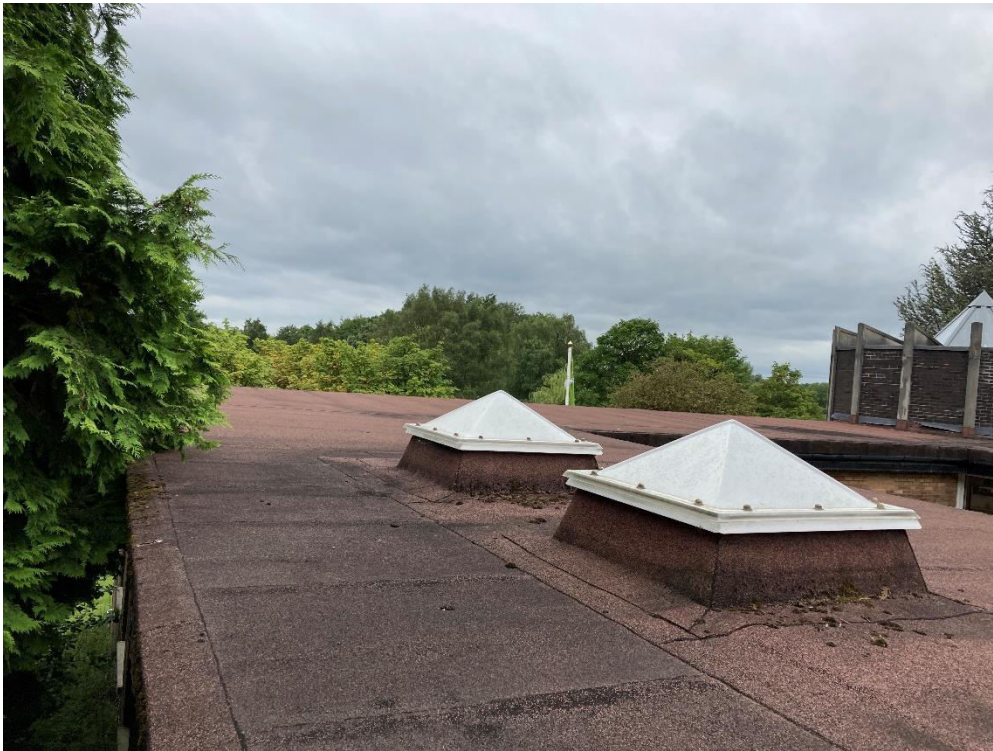
Image 03: Office & Yard Flat Roof Covering and Rooflights
