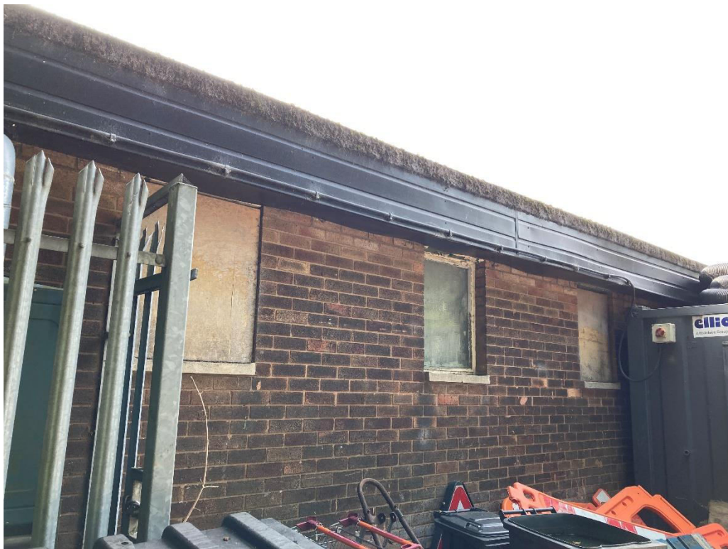
Image 02 – Ladder Access Location Nr.1
