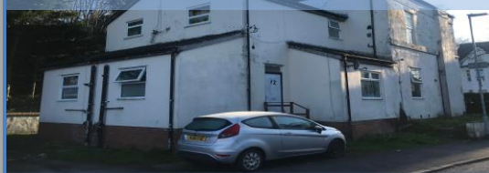
The Moxley Road elevation of number 27 and the rear elevations of both properties
