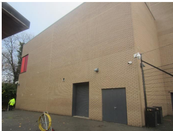
Photo 11: Southern elevation of the school building to be extended
