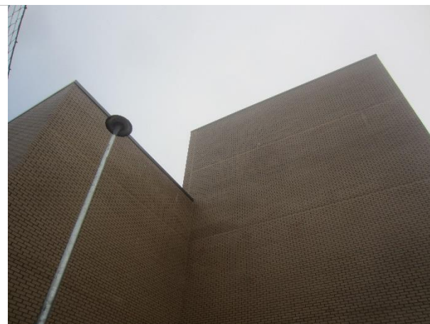
Photo 12: Southern elevation of the school building to be extended
