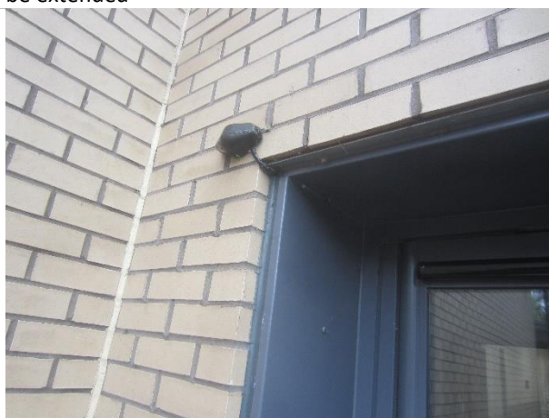
Photo 13: No gaps or potential roost features around doorways at southern end of school building
