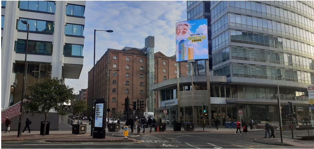
Plate 2: View looking ENE towards Ducie Street from Auburn Street, with the digital advertisement attached to the corner of Gateway House visible alongside the Grade II listed London Warehouse
