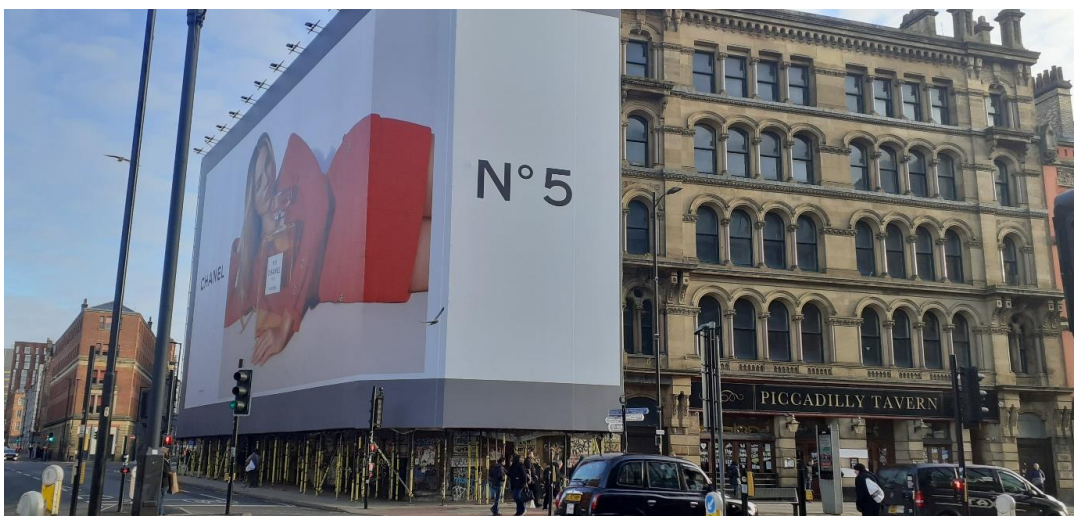
Plate 3: View NE from Piccadilly towards the large-scale advertisement at No. 67, at the corner of Piccadilly and Newton Street, with the Grade II listed buildings at Nos. 69-75 visible to right of picture
