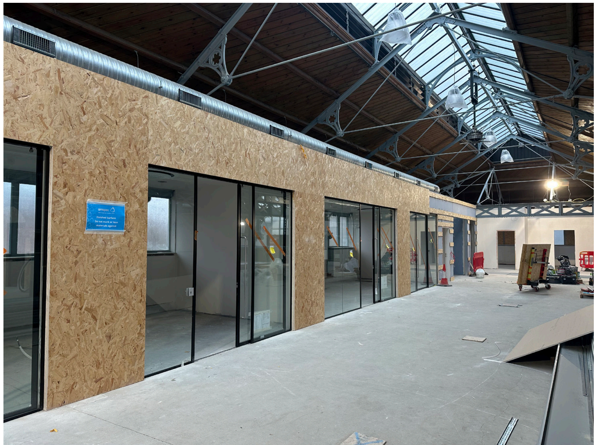
OSB Finish to Perimeter Mezzanine Worksuites
