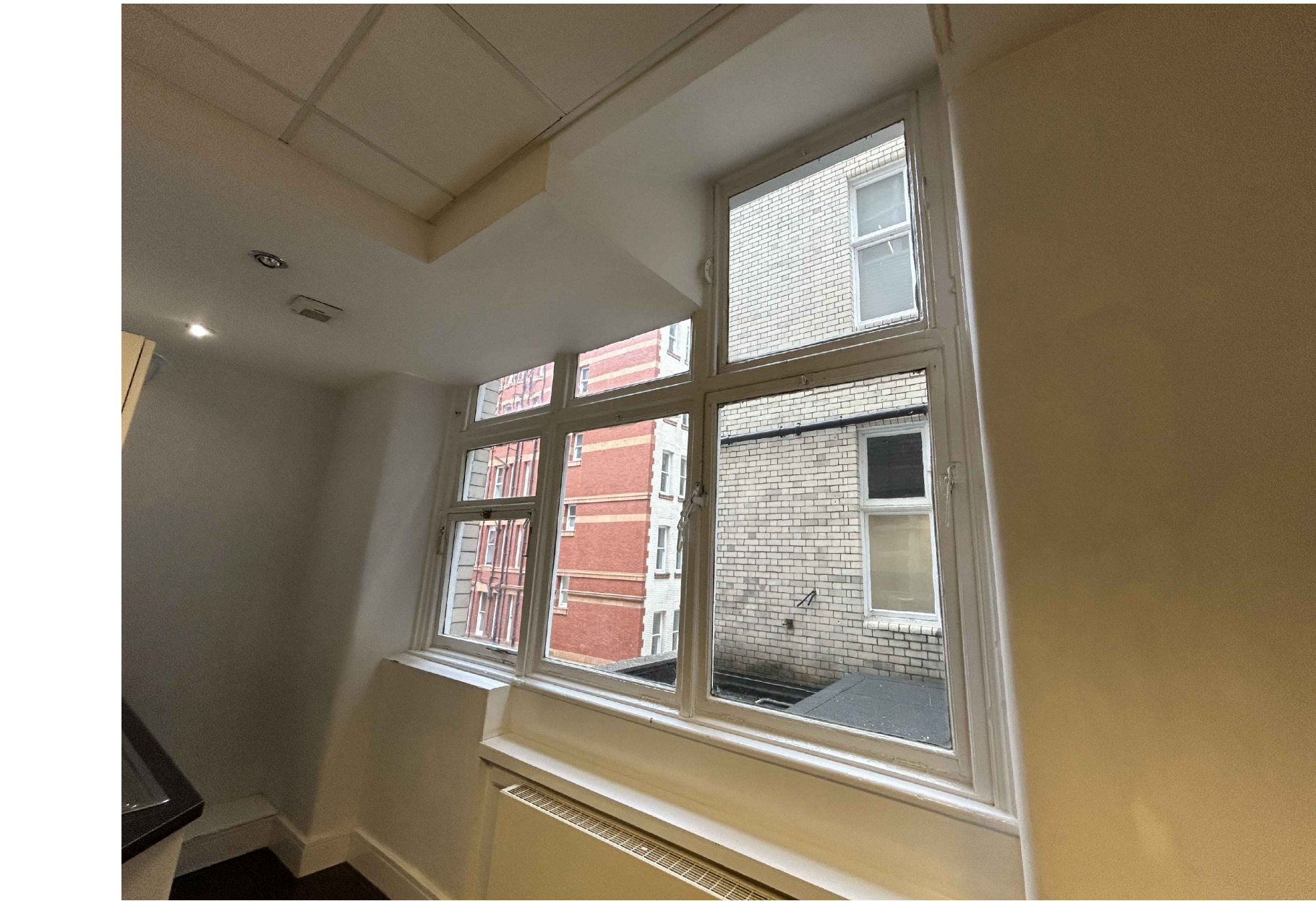
02 WINDOW TYPE 6 EXISTING PHOTO 556 SCALE - NTS PHOTO
