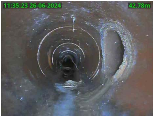
MH 8301X_c62f1032-655e-40e3-b64c-382543fe9a78_20240626_1 45043_752.jpg, 00:03:10, 42.78 m Connection other than junction at 3 o'clock, 150mm dia
