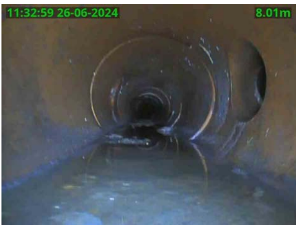
MH 8301X_142bd1e8-ace7-47c7-bdfa-450c50568fd0_20240626_1 44218_195.jpg, 00:00:46, 8.01 m Junction at 3 o'clock, 150mm dia
