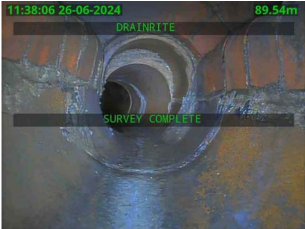
MH 8301X_245511b9-d425-449c-9e82-7af805317fe1_20240626_145849_728.jpg, 00:05:53, 89.54 m Finish node, manhole, reference: MH 8301
