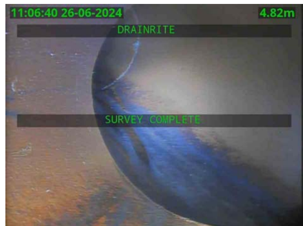
MH F1X_c3397df3-4d91-4727-aa5e-cf349abf8ae6_20240626_150 334_906.jpg, 00:01:39, 4.82 m Finish node, manhole, reference: MAIN
