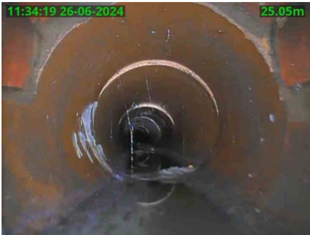
MH 8301X_5f8237f5-9584-41bc-8471-d31ab0e967a0_20240626_1 44711_189.jpg, 00:02:06, 25.05 m Pipe size changes, new size(s), 300mm high
