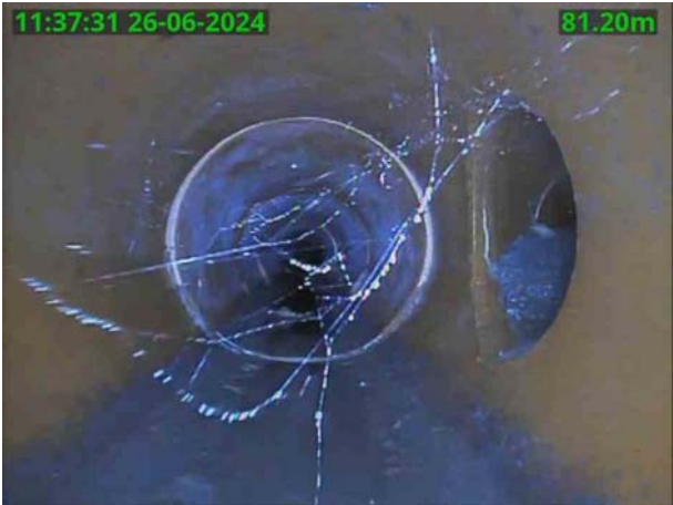
MH 8301X_3881f1fd-5daf-41cb-85b6-0ad9ba793248_20240626_145755_496.jpg, 00:05:18, 81.20 m Junction at 3 o'clock, 150mm dia
