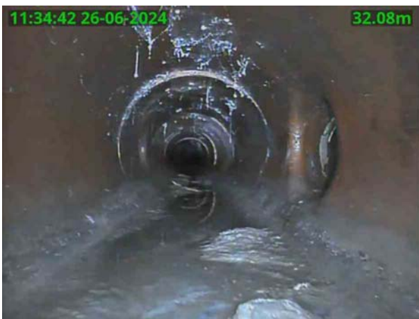
MH 8301X_4c0a1c7c-b223-409e-a920-30bd46e6bb73_20240626_ 144835_838.jpg, 00:02:29, 32.08 m Junction at 3 o'clock, 150mm dia
