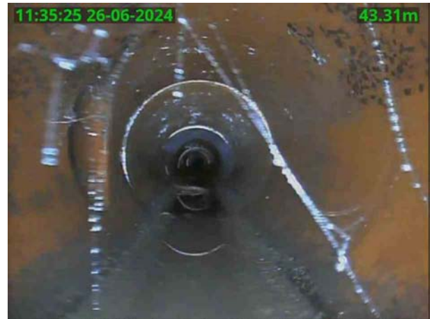
MH 8301X_1a69736d-cd99-4ada-a9fc-5bb92a38fcf8_20240626_1 45111_172.jpg, 00:03:12, 43.31 m Junction at 9 o'clock, 150mm dia
