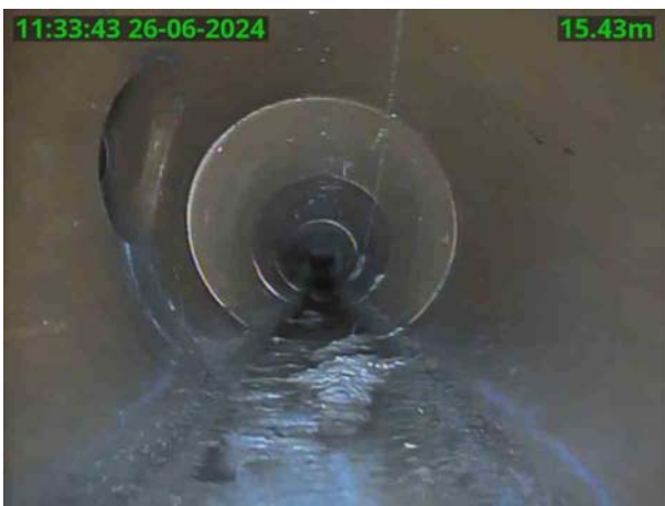
MH 8301X_9846d641-6b70-48dd-9cdb-c5113f770cc4_20240626_ 144455_462.jpg, 00:01:30, 15.43 m Junction at 9 o'clock, 150mm dia
