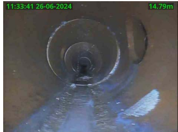
MH 8301X_4e61f0c1-8992-4472-8420-84c78c71e576_20240626_ 144427_700.jpg, 00:01:28, 14.79 m Junction at 3 o'clock, 150mm dia
