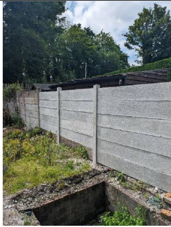
Photograph 4: West aspect of the site with a concrete fence, scattered scrub/ oriental plants and a brick ditch (TN-2)..
