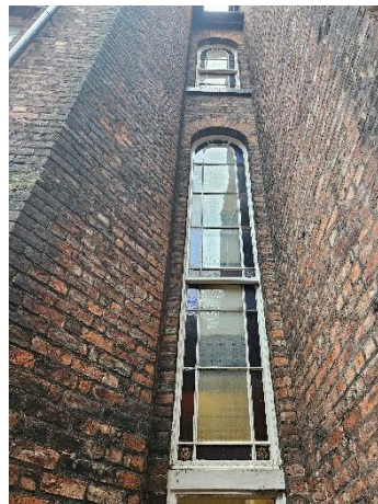
Figure 11: Rear Window Detail
