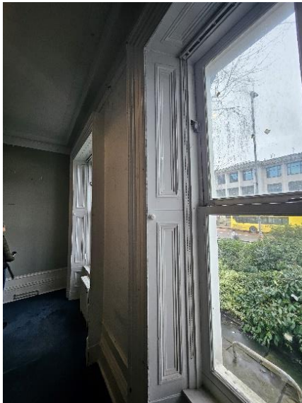
Figure 18: View onto Oxford Rd. Halliday Meecham Architects
