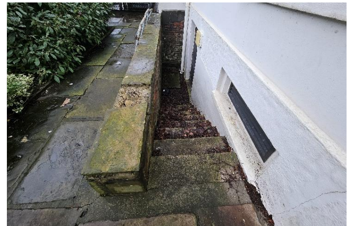
Figure 13: Basement Steps to front entrance
