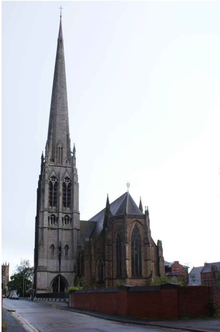
Fig. 23.) St Walburge's, Preston (James Crowley 2020)
