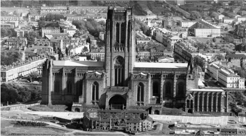
Fig. 25.) Aerial view of Liverpool Anglican Cathedral in 1987 (© liverpoolecho.co.uk)
