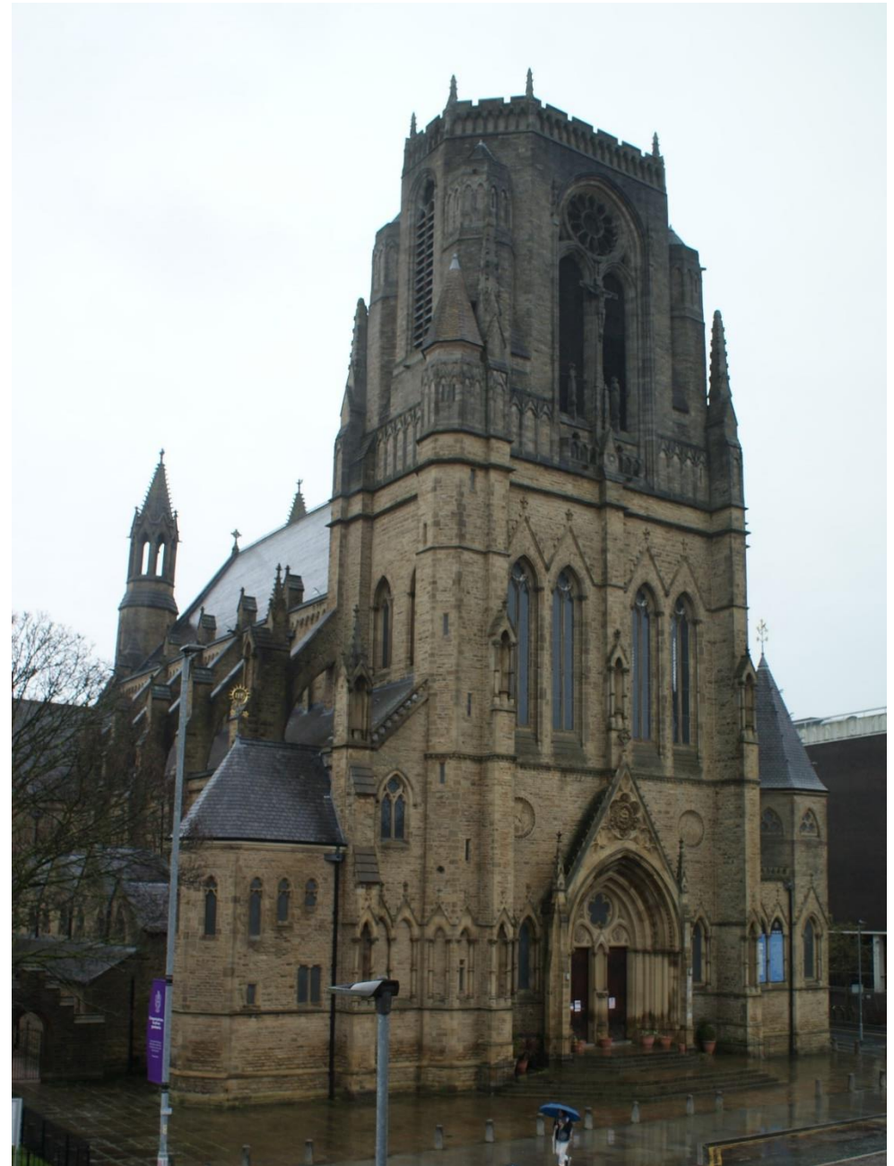
Fig. 29.) The west front and tower (James Crowley, 2023)
