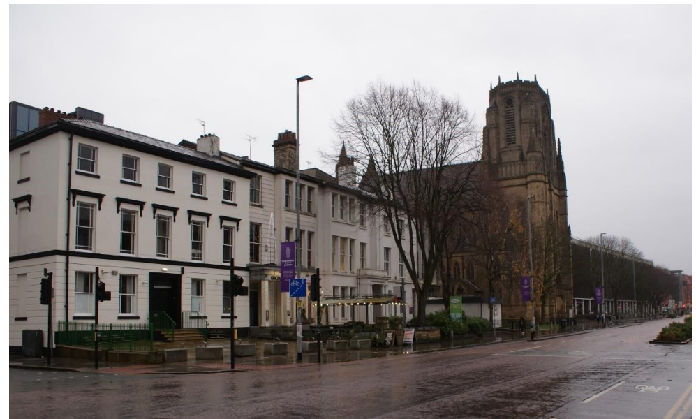
Fig. 6.) The church as seen from Oxford Road (James Crowley, 2023)
