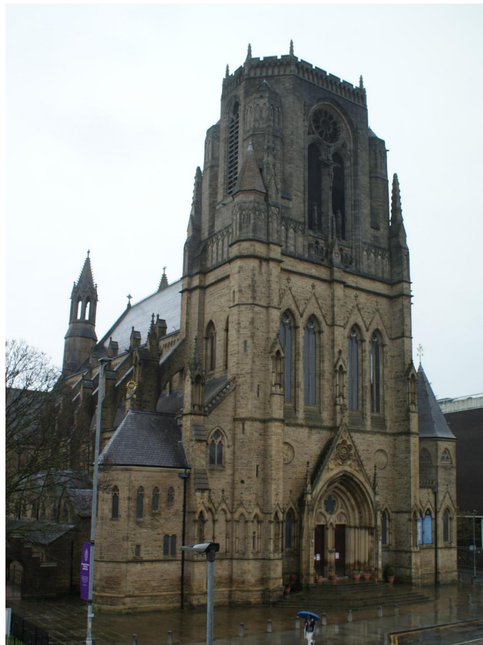
Fig. 7.) The west front and tower (James Crowley, 2023)
