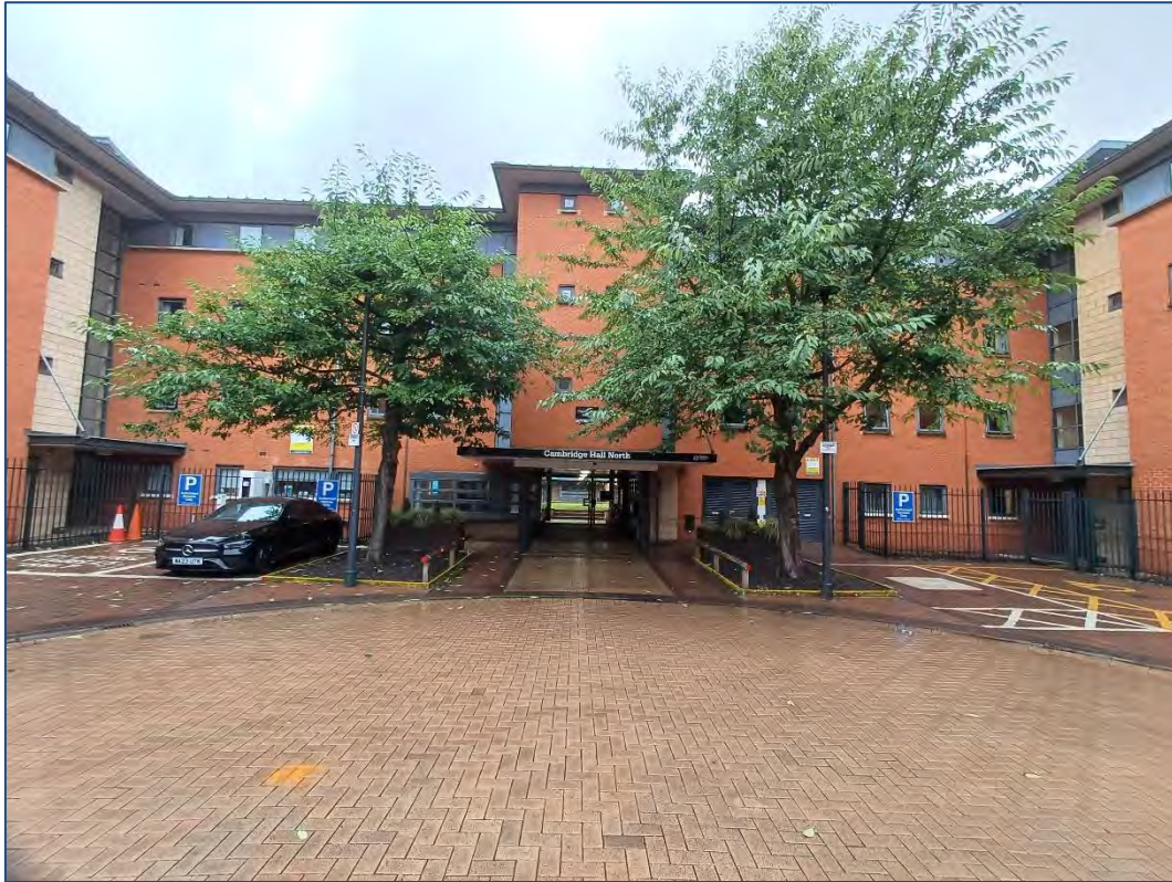
Plate 9: View across southeastern façade of Cambridge North Building, from the southeast
