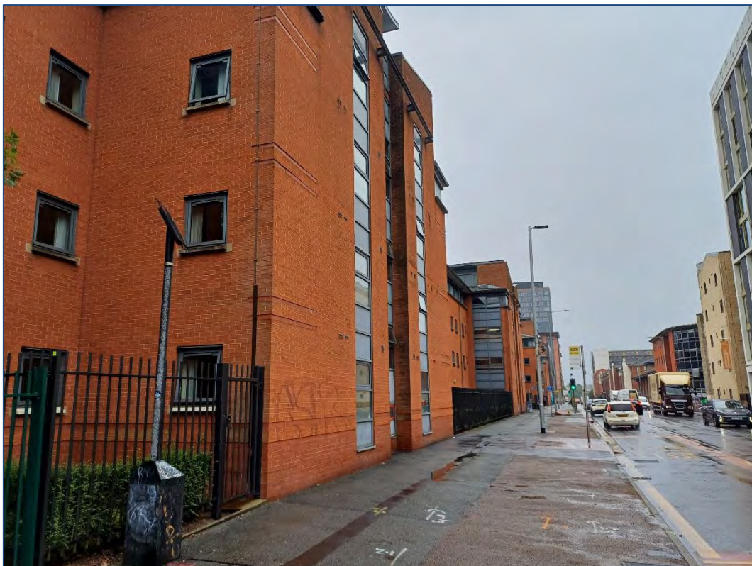
Plate 10: View across southwestern façade of Cambridge North Building, from the northwest
