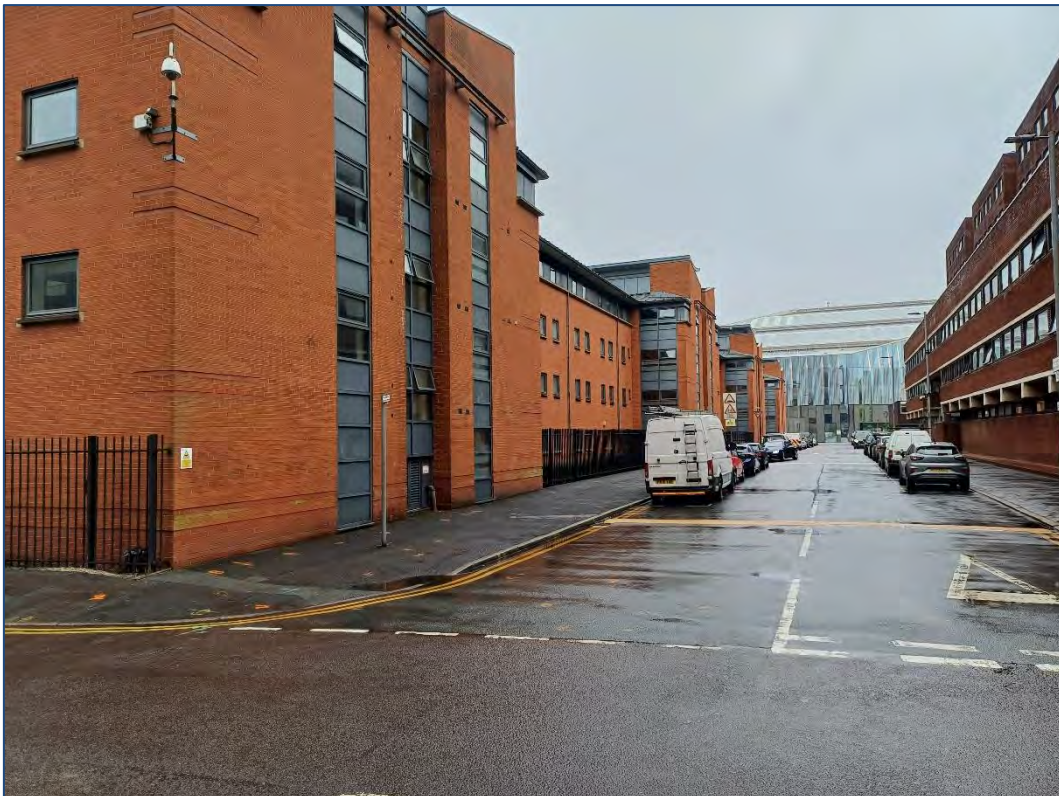
Plate 12: View across northeastern façade of Cambridge South Building, from the east
