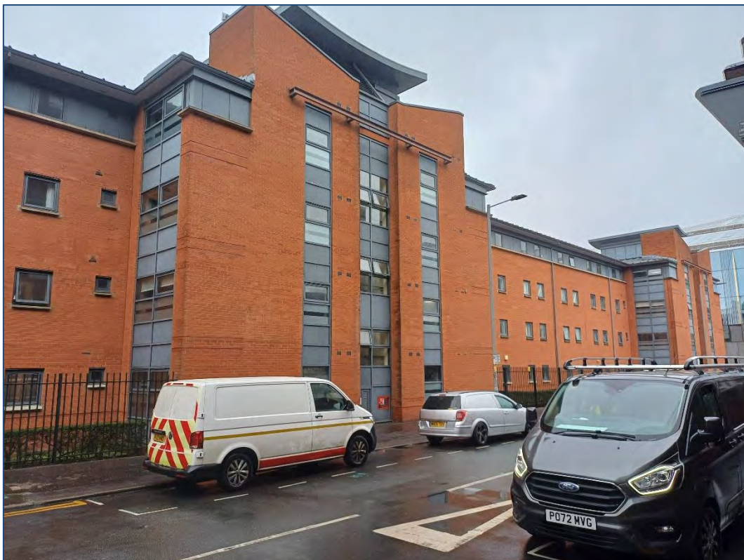
Plate 8: View across northeastern façade of Cambridge North Building, from the east
