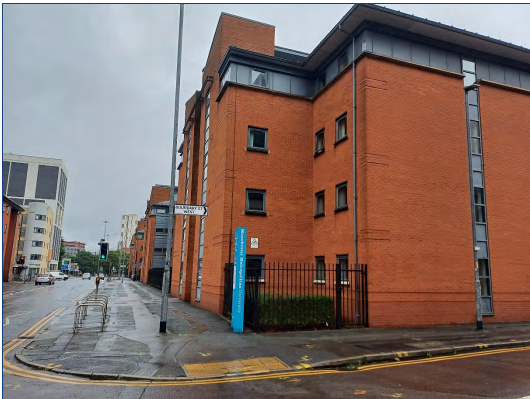
Plate 14: View across southwestern façade of Cambridge North Building, from the southeast
