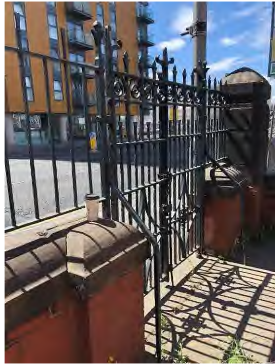
Figure 35: The reused 19 th century stone copings, gates and pier to the west of the boundary wall.
