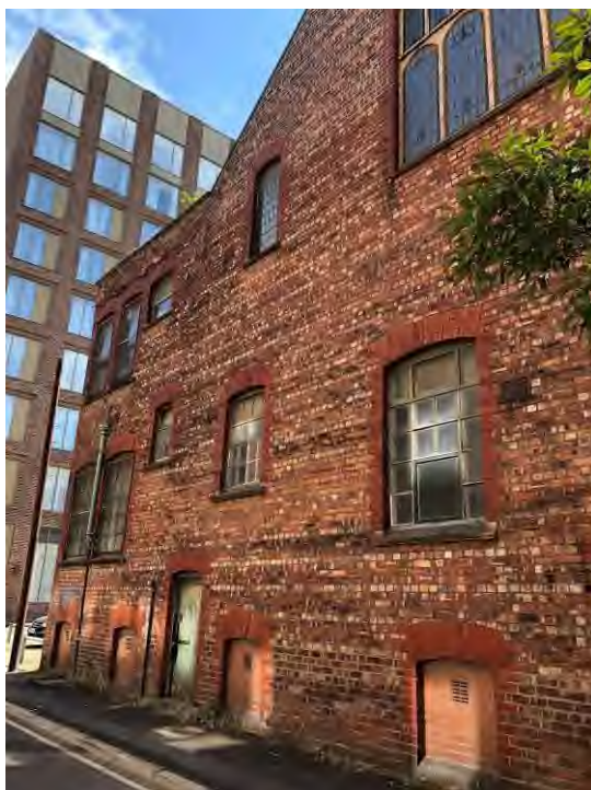
Figure 42: The rear, north elevation on Dyche Street.
