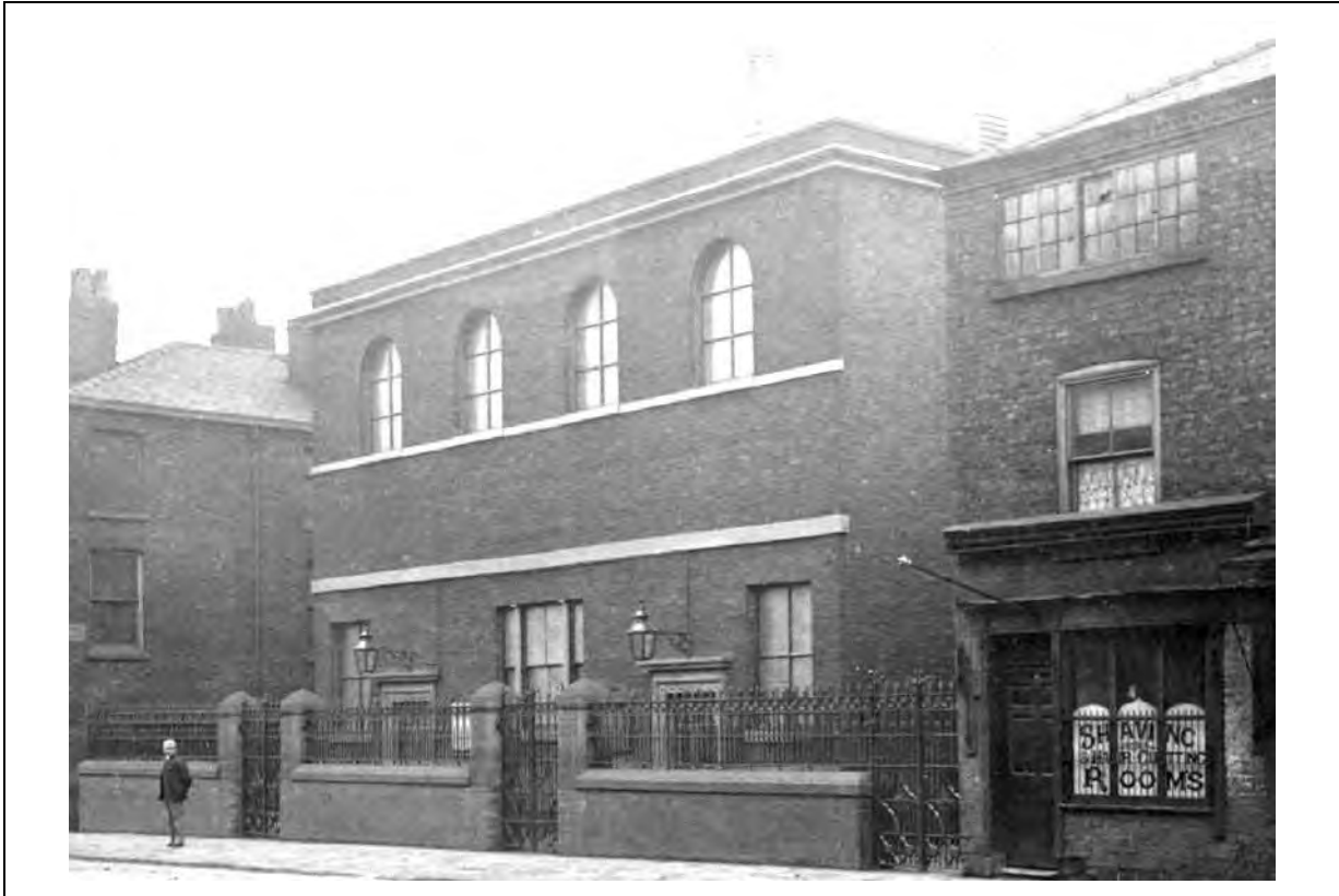
Figure 11: The south elevation of the c1823-4 chapel as seen in 1900, showing the replacement of the original sash windows with fixed windows (Source: Manchester Archives)
