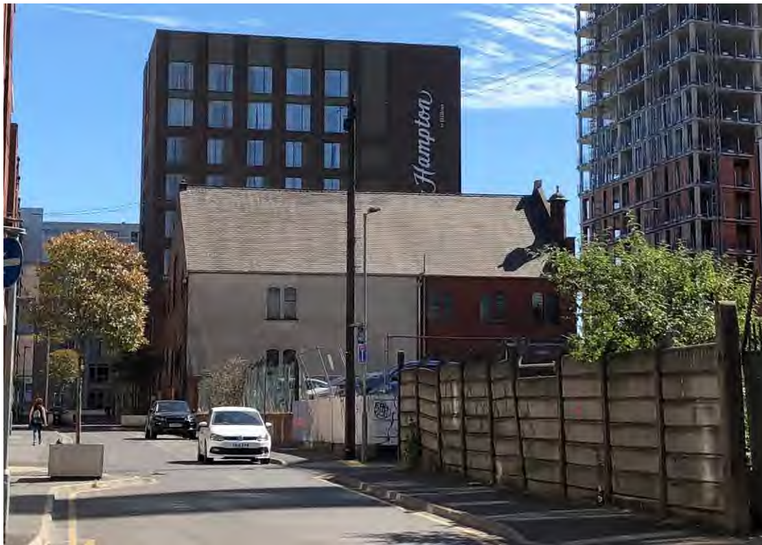
Figure 41: Looking east along Dyche Street towards the west elevation of the chapel, illustrating the scarring resulting from previous buildings since demolished.
