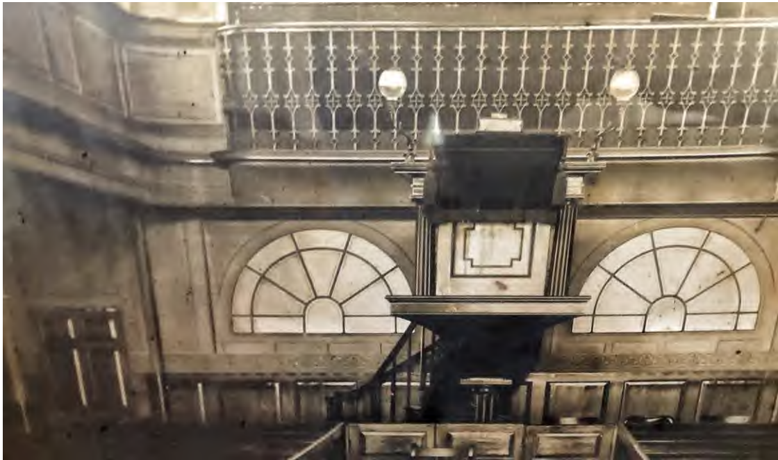
Figure 14: A closer 1906 view of the original c1823-4 pulpit, cast iron railings and panelled balcony, which were all reused in the current building. (Source: Particular Baptist Chapel)
