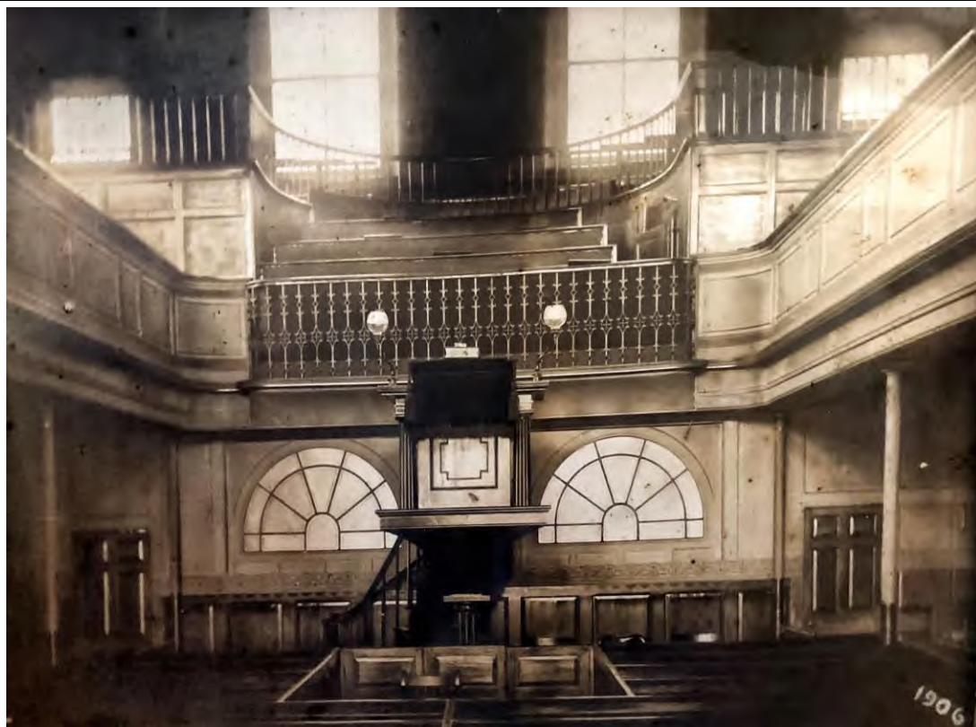
Figure 13: 1906 photograph looking north towards the original c1823-4 pulpit, as used by Rev William Gadsby (Source: Particular Baptist Chapel)
