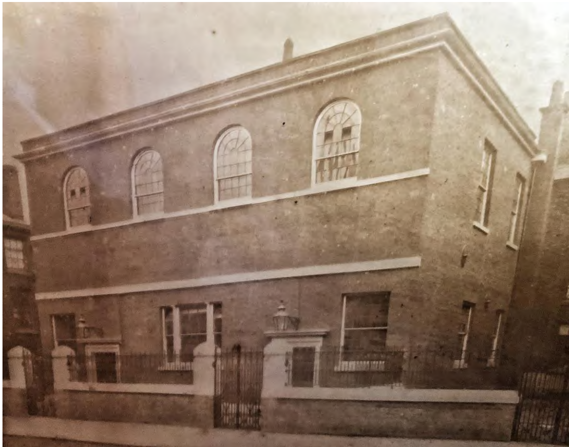
Figure 9: c1860s-80s photograph of the south entrance front of the original chapel, showing its early-19th century southern elevation. Note the original wall copings/piers and 19 th century gates, which still survive today (Source: Particular Baptist Chapel)
