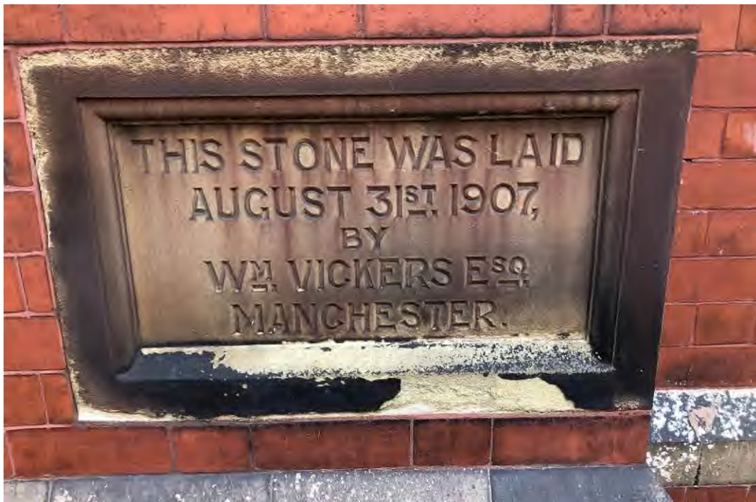
Figure 40: The original foundation stone to the south elevation, placed here on the 31 st August 1907 by William Vickers Esq.
