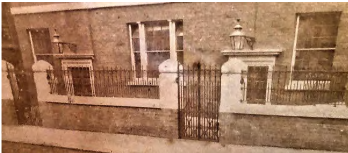
Figure 10: Detailed c1860s-80s view of the early 19 th century grit stone wall copings, gate piers and 19 th century cast iron railings/gates, which were reused in the current boundary wall (Source: Particular Baptist Chapel)
