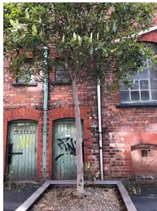
Figure 43: The rear, north elevation on Dyche Street, showing the original basement storage room doors.
