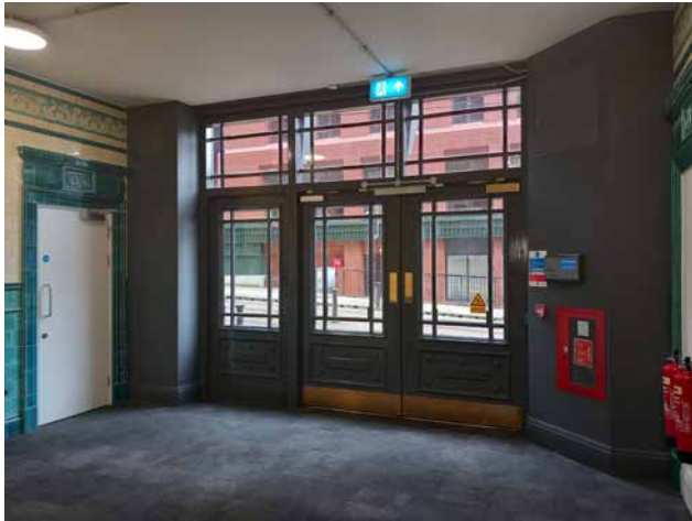
3.29 Hanover Building, Bloom Street staircore - entrance
