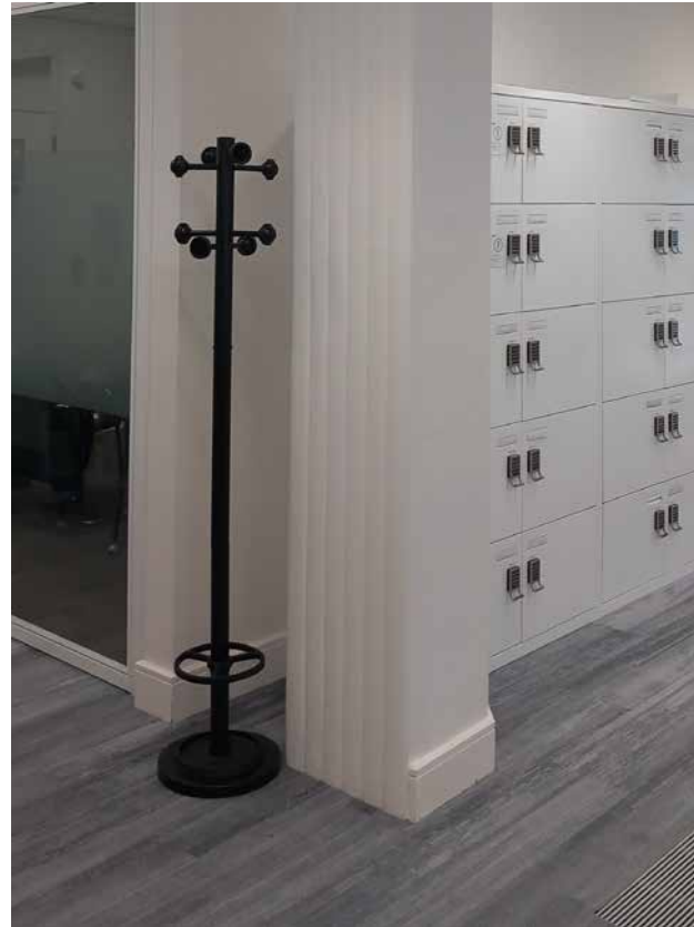
3.52 1 st floor, Hanover Building - 1930s fluted column
