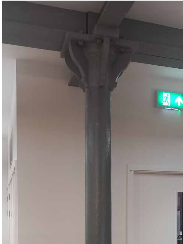
3.46 1 st floor, E Block - beams, column and capital
