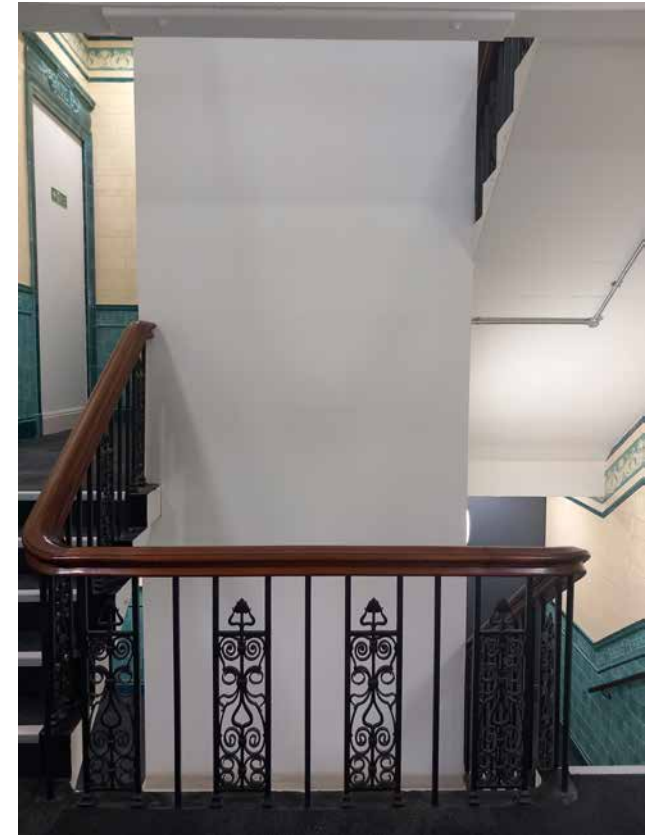
3.32 Hanover Building, Bloom Street staircore - lift
