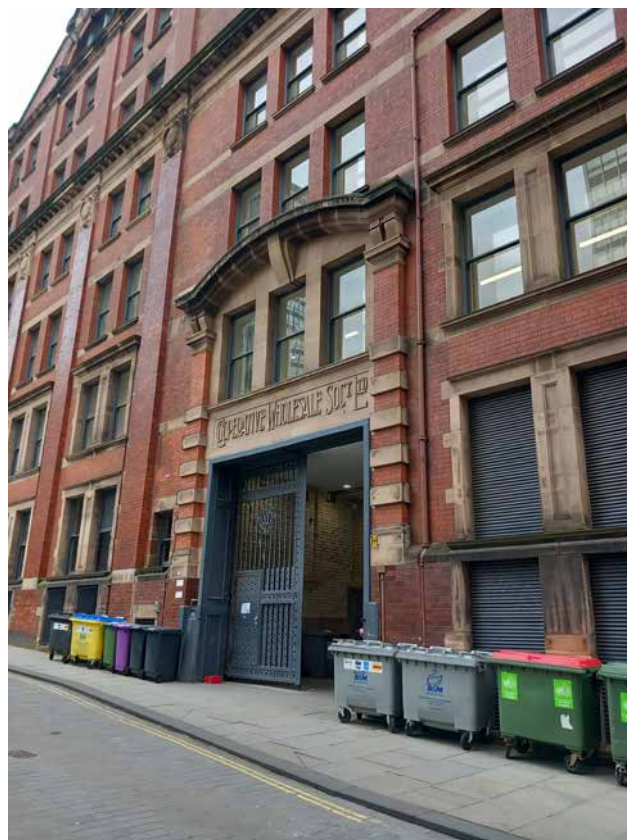
3.21 E Block - Hanover Street loading entrance
