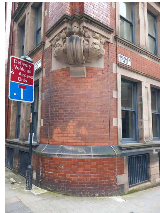
3.22 E Block - Federation Street - Hanover Street sandstone carving
