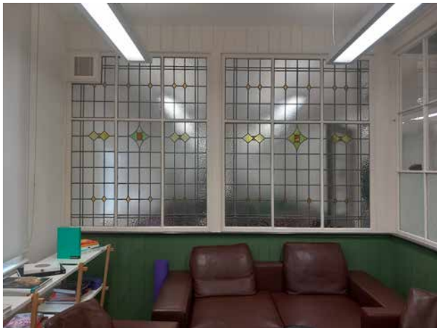
3.45 1 st floor, E Block - timber screens forming offices with leaded lights
