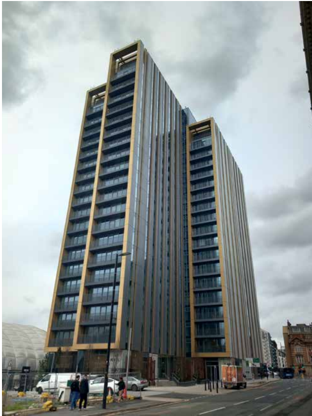
3.2 Facing side of Corporation Street
