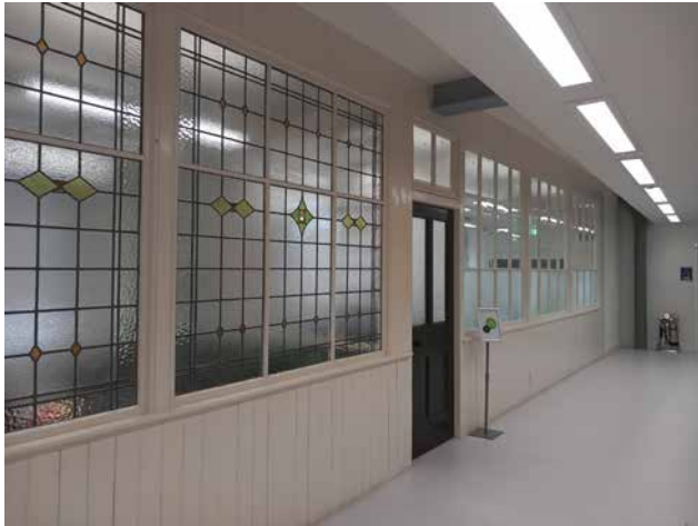
3.44 1 st floor, E Block - timber screens forming offices
