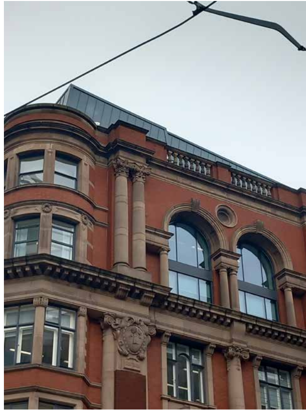
3.16 Hanover House - contemporary attic windows and roof extension
