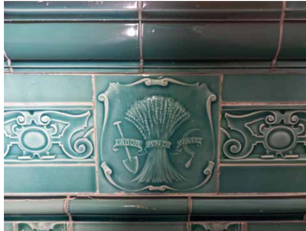
3.34 Hanover Building, Bloom Street staircore - CWS emblem
