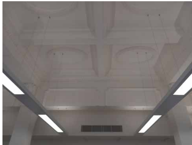
3.56 2 nd floor, Hanover Building - 1930s decorative ceiling and M+E suspended ceiling
