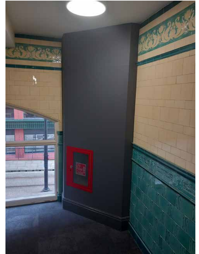
3.35 Hanover Building, Bloom Street staircore - service riser
