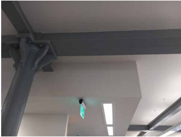
3.47 1 st floor, E Block - M+E suspended ceiling
