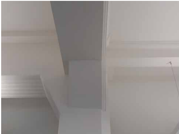
3.53 1 st floor, Hanover Building - beams and column heads
