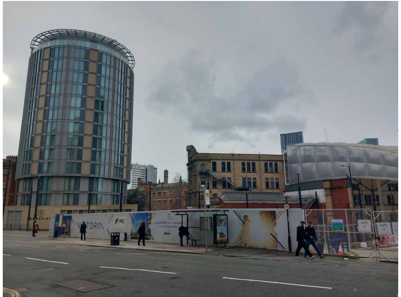
3.1 Facing side of Corporation Street including Victoria Station
