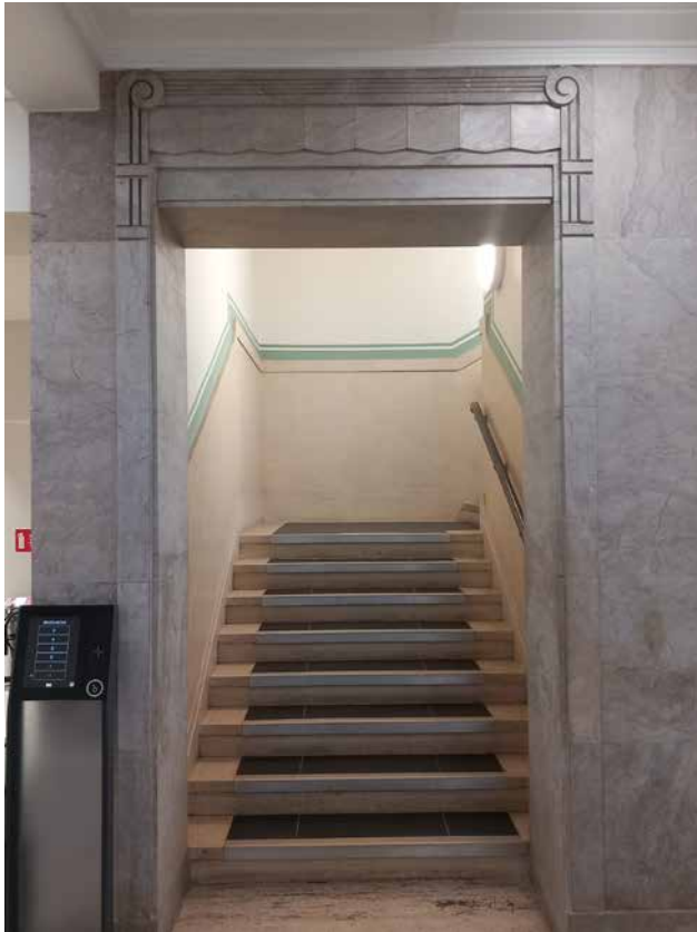
3.26 Hanover Building, central staircore - reception entrance
