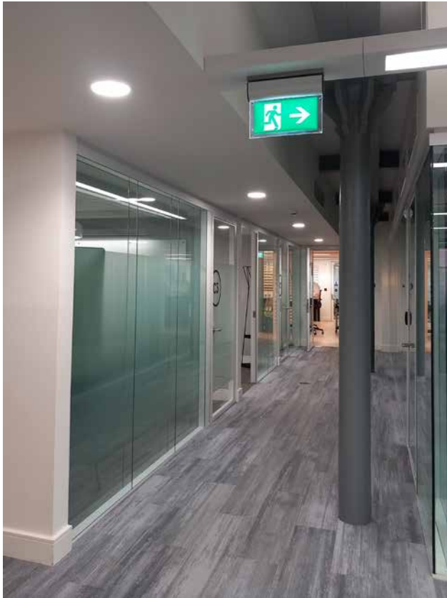
3.54 2 nd floor, E Block - office partitions, exposed structure and M+E suspended ceiling
