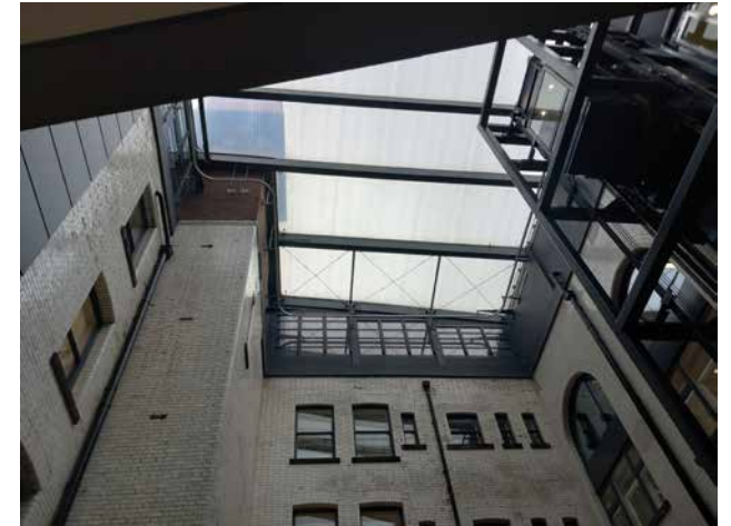
3.25 Atrium - contemporary roof
