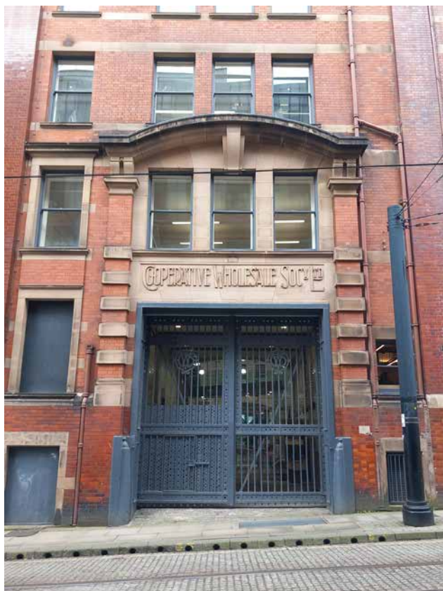
3.20 E Block - Bloom Street loading entrance
