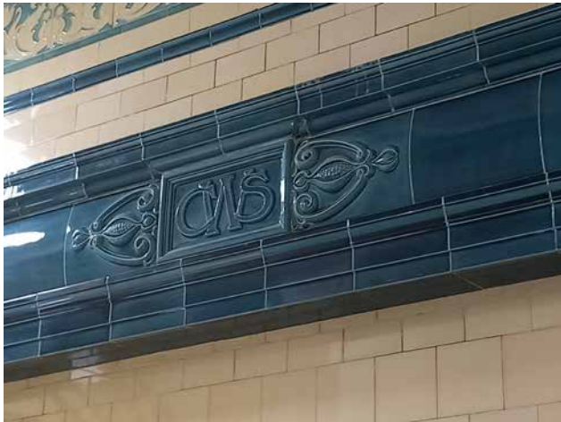
3.30 Hanover Building, Bloom Street staircore - CWS dado emblem
