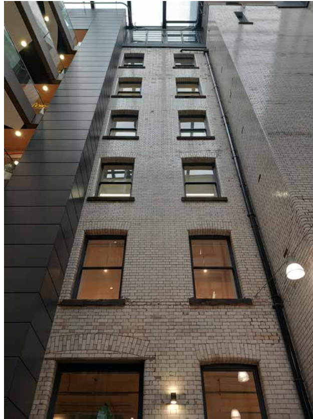
3.24 Atrium - one-over-one sash windows and contemporary service riser
