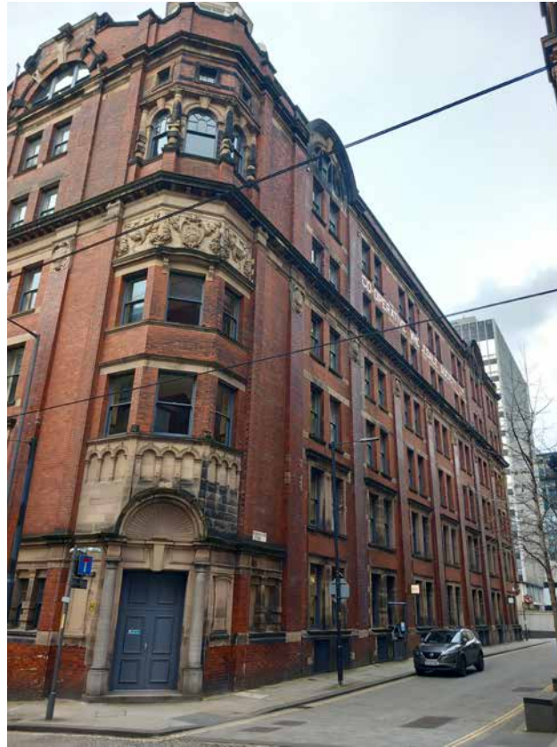
3.18 E Block - Federation Street facade and public entrance
