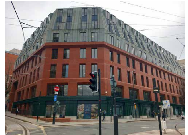
3.8 Late-20 th century six-storey Co-Operative Bank office block
