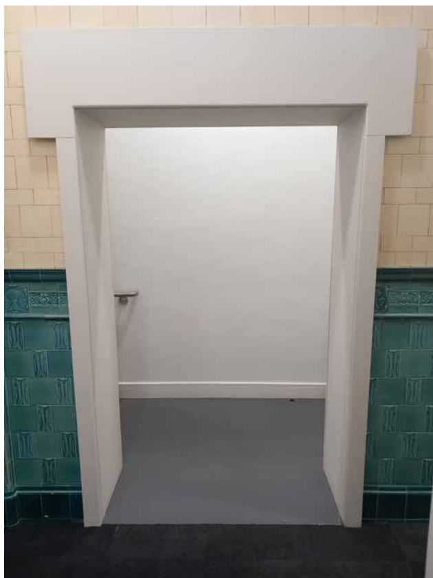
3.39 Hanover Building, Hanover Street staircore - opening
