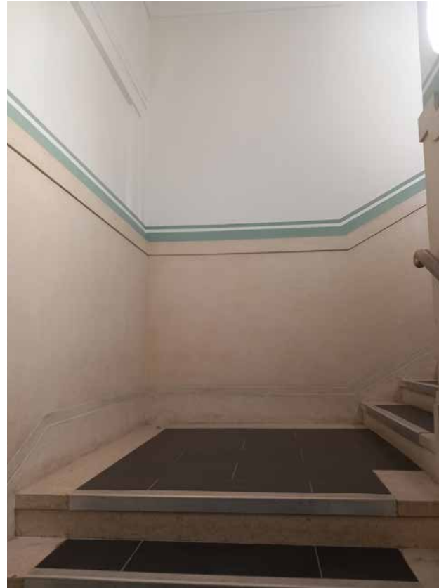
3.27 Hanover Building, central staircore - terrazzo finish
