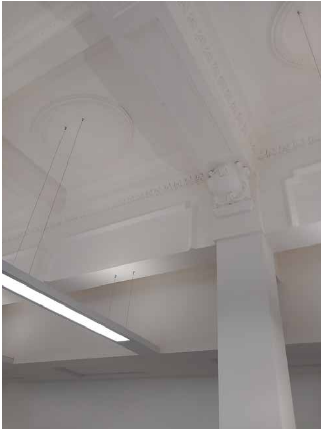
3.57 2 nd floor, Hanover Building - 1930s decorative capital
