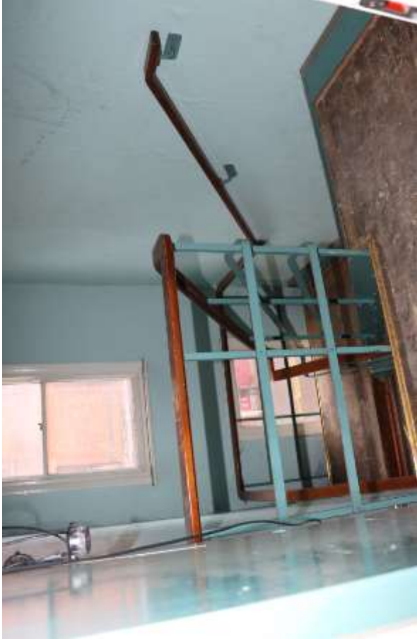
Photograph 40. Looking down from the second floor staircase landing in the rear part of the building.
