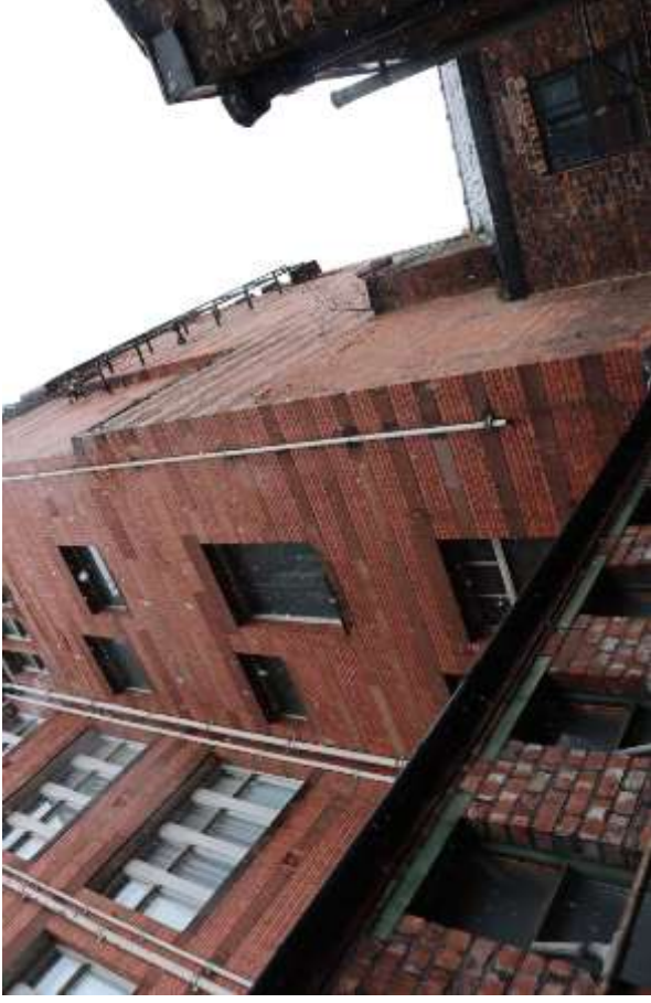
Photograph 18. A view from the flat roof at first floor level.
