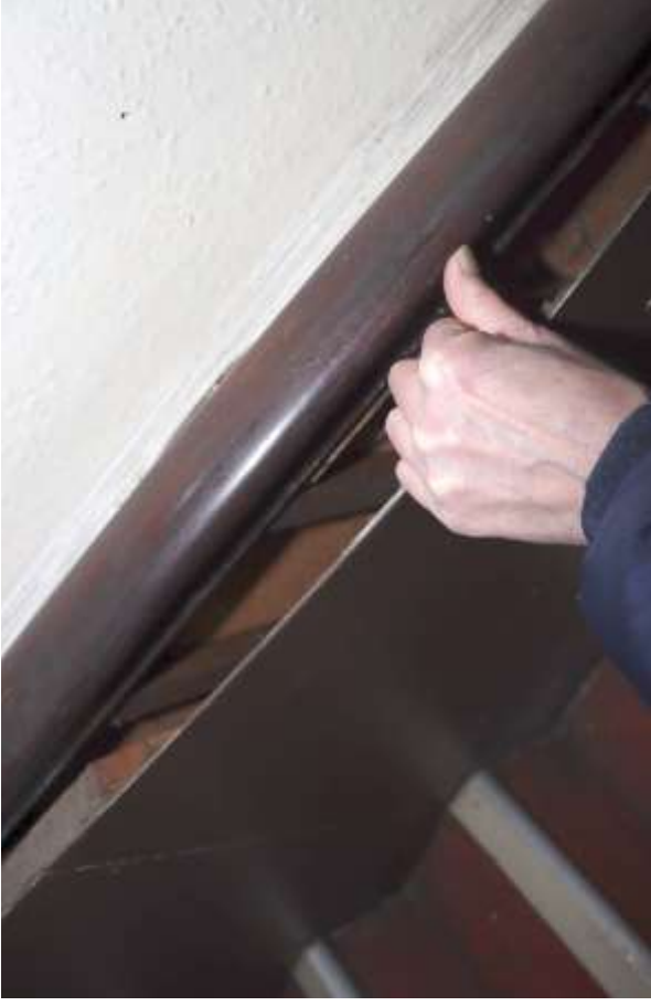
Photograph 22. The balustrade to the staircase that leads from behind the bar in the pub to the first floor.
