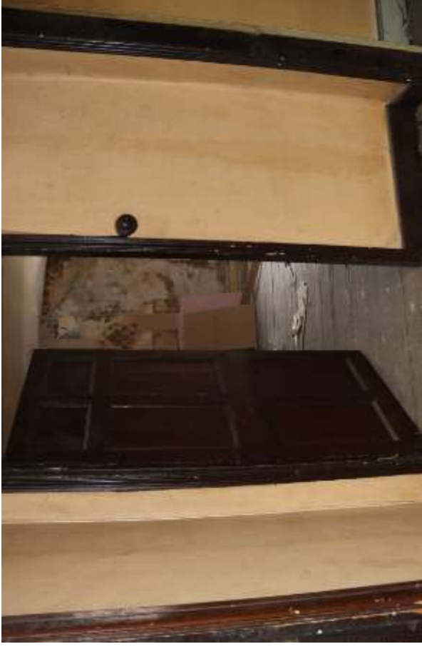
Photograph 30. A 6-panel door on the second floor.
