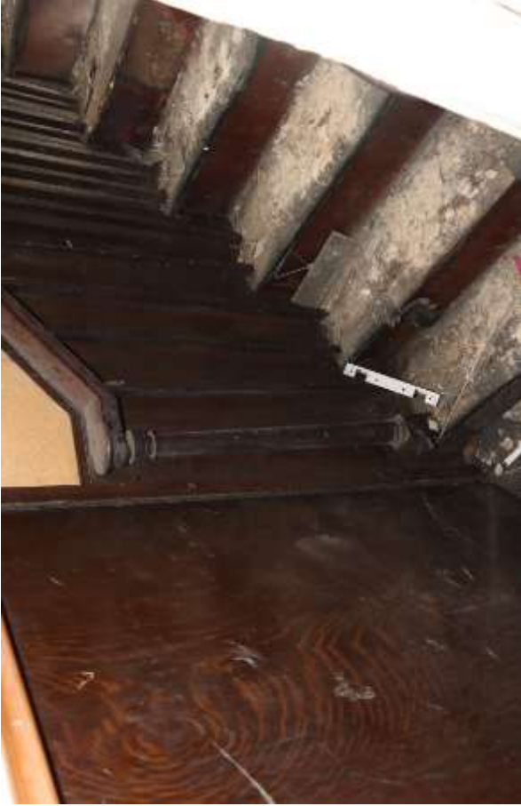
Photograph 25. The staircase from the first to the second floor in the front part of the building.
