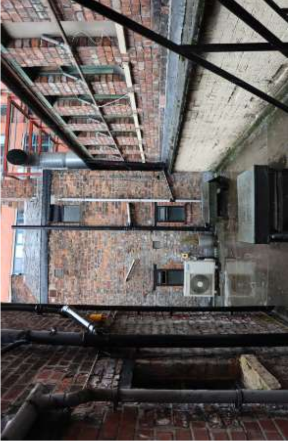
Photograph 14. Looking towards the rear from a first floor window.
