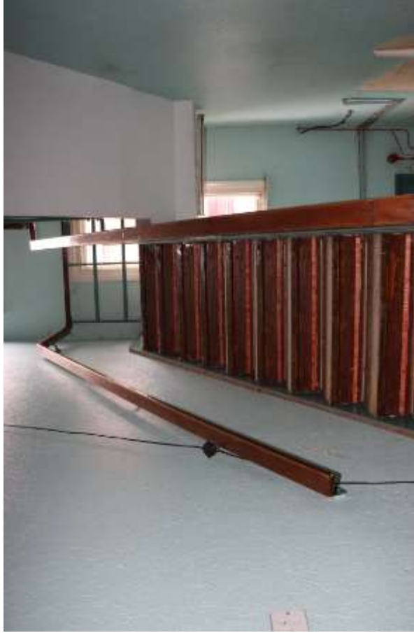
Photograph 35. The staircase from the first to the second floor in the rear part of the building.
