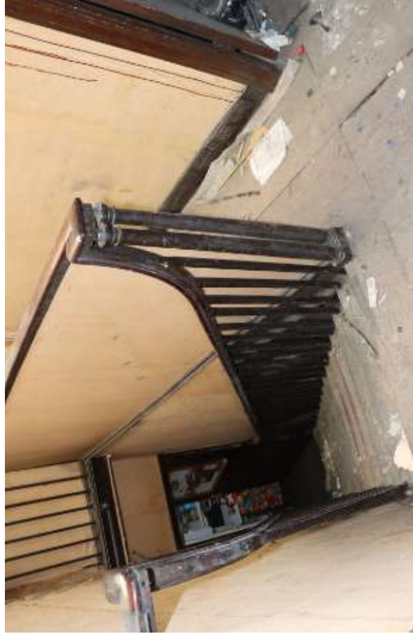
Photograph 27. The staircase from the first to the second floor in the front part of the building.
