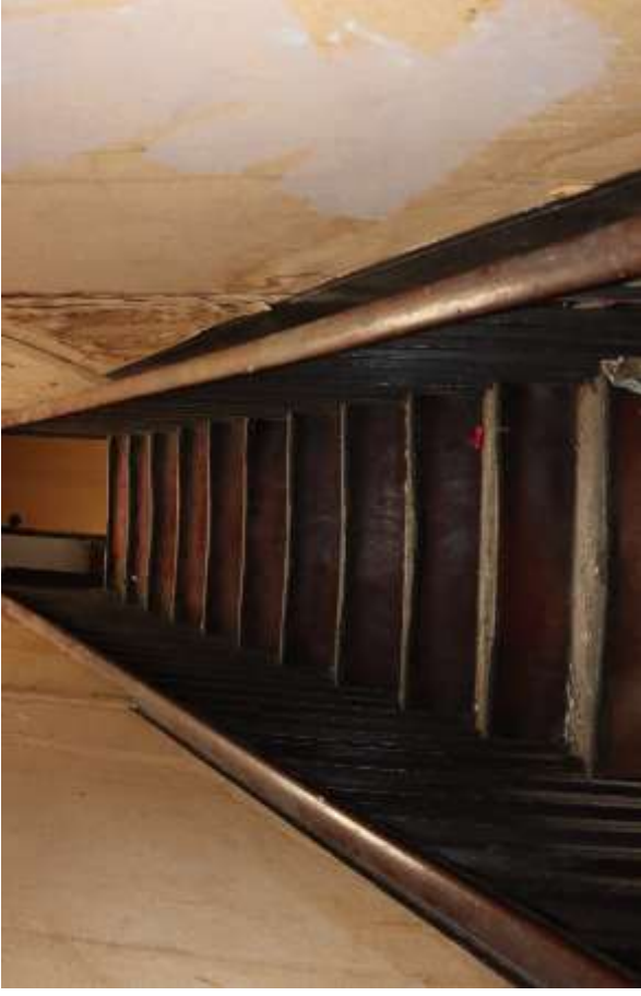
Photograph 26. The staircase from the first to the second floor in the front part of the building.
