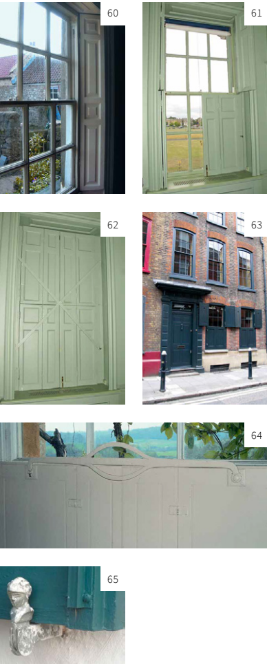
60-62. Double hung sash windows with internal shutters which fold into recesses on each side of the window. When fully closed the shutters are secured tightly with iron shutter bars. 63. External shutters from the 18th -century divided into upper and lower leaves to give greater flexibility in balancing requirements for light, ventilation and security. 64. These internal shutters which are divided horizontally have a security bar which locks the lower panels in place. 65. A holdback for external shutters.
