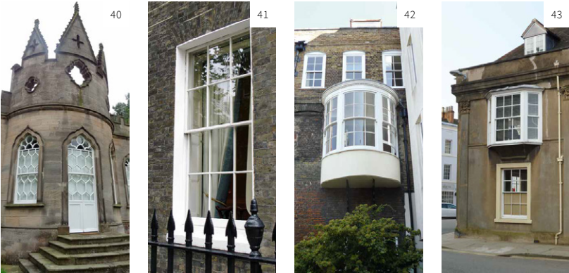
Images 40-43 40. Elaborate mid-18th-century ‘Gothick’ windows. 41. In 1774, further legislation in London led to sash boxes being hidden within a rebate formed in the brickwork surrounding the window opening. This, combined with very slender glazing bars gave windows a much lighter and more delicate appearance.
