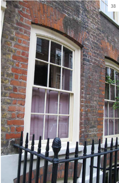
Images 38 and 39 38. In the cities of London and Westminster, legislation came into force in 1709 which required window frames to be set back from behind the wall face.
