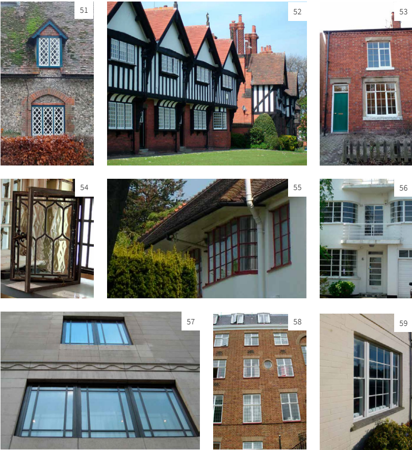
Images 51-59 51. Cast iron windows in a lattice pattern were used widely for estate cottages in the mid 19th-century and many still exist. 52-53: Small pane cottage windows became popular towards the end of the 19th century for model workers housing as shown here at Port Sunlight and New Bolsover. 54. Early 20th-century Crittal window dating from 1904 (from the Brooking Collection). 55. Steel windows became a feature of inter-war suburbia. 56. 1930s 'Modern Movement' style steel windows with balcony railings. 57. During the inter-war years non-ferrous metals such as bronze started to be used for windows largely for the non-domestic market. 58. Steel windows combined with leaded lights in a block of 1930s flats. 59. A rare three light steel sliding sash window dating from the early 1950s.
