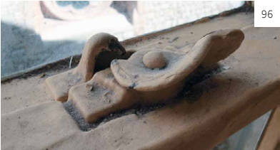
Images 95 and 96 95. In a double hung sliding sash window each sash has its own pulley and cord. The parting bead separates the sashes and holds them in position. The cord and pulley need to be kept in good working order. 96. A Fitch pattern sash fastener.
