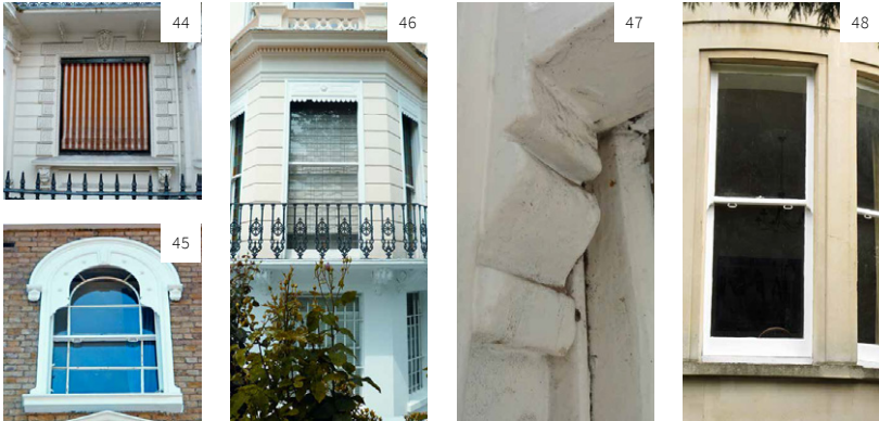
Images 44-48 44. A rare surviving awning. 45. Remains of cases for external blinds and awnings still exist on some Victorian buildings. 46. Bay windows have foundations and may be one or several storeys high. 47 & 48. In the late 19th-century vertically sliding sash windows began to make use of larger and heavier panes of glass. The weight of the glass, coupled with the disappearance of the glazing bars that had given support to the horizontal meeting rails, led to the development of ‘horns’ which strengthened the joint between the meeting rail and the stiles.
