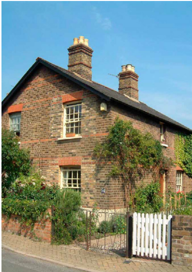
Image 140 Windows of the original size and pattern have been reinstated in this south London conservation area which has involved reinstating the original masonry openings.
