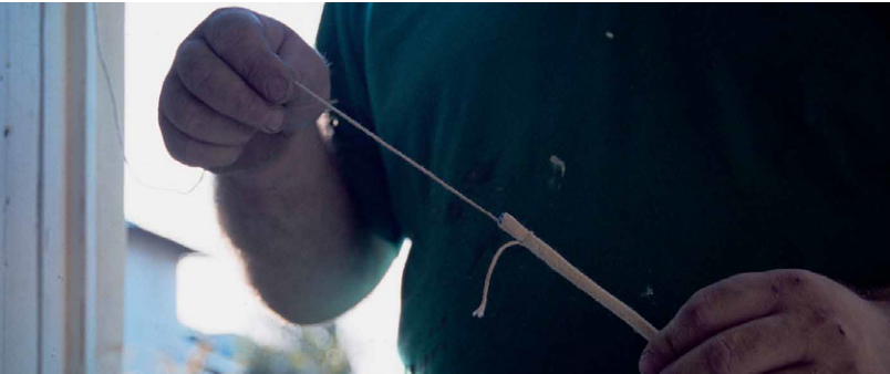
Image Tying a lead ‘mouse’ and string to the new sash cord.
