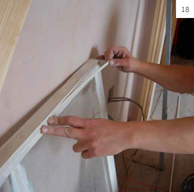
Images 18 and 19 The thermal performance of single glazed traditional windows can be improved significantly by draught-proofing or secondary glazing.
