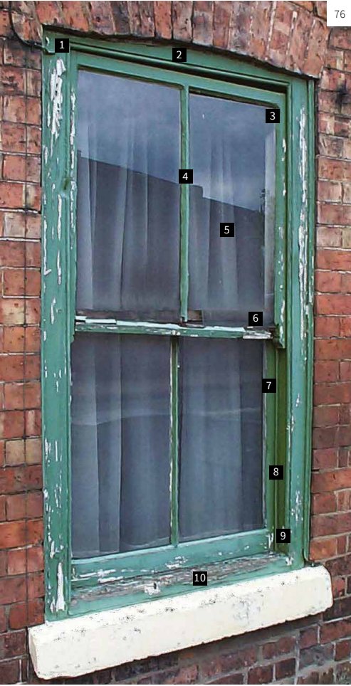
Key to Image 76 1. Holes drilled in frame for cable entry may admit water and cause decay. 2. Deformation of window caused by structural movement in wall; sashes no longer fit or slide properly. 3. Broken sash cords. 4. Breakdown of paint and putty caused by lack of regular maintenance; this allows water to penetrate and become trapped, causing decay. 5. Glass displaced or broken due to deformation of sash. 6. Failure of joints, caused by timber decay due to water penetration. 7. Opening parts of window jammed due to accumulation of paint. 8. Worn or damaged beads, causing rattles and draughts. 9. Decay of stile (or jamb) and outer lining at junction with cill due to water penetration. 10. Decay of cill caused by water penetration after breakdown of paint. Water may also creep into the joint between the timber cill and the masonry sub-cill.
