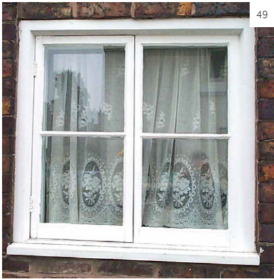
Images 49 and 50 49. A simple 19th-century timber side-hung casement window. The uniformity of the frame proportions is maintained by the split mullion.
