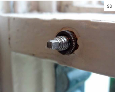
Images 97 and 98 97. Height restrainers allow a degree of ventilation without compromising security. 98. Bolts inserted into the meeting rails of a sash window keep the two sashes firmly locked in place.
