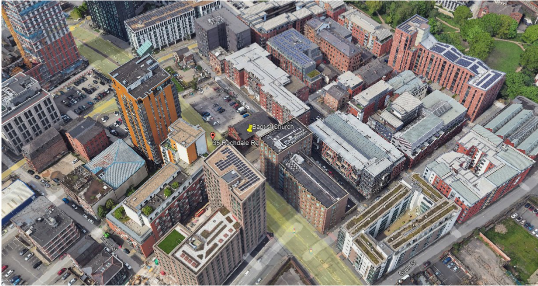
Figure 12.2 – Existing Site for Baseline Assessment
