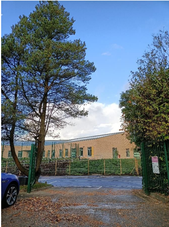
Figure 2.3: Site entrance from Crescent Drive.
