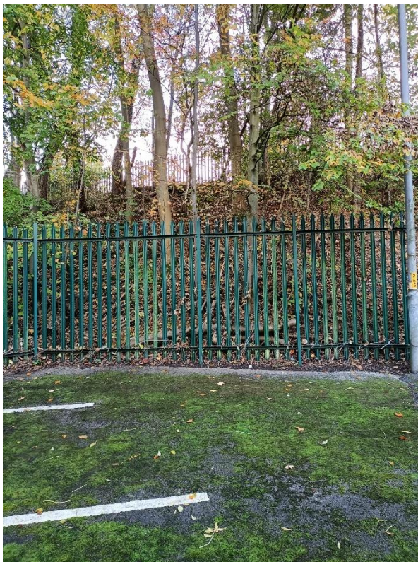
Figure 2.5: Slope adjacent to the eastern car park.
