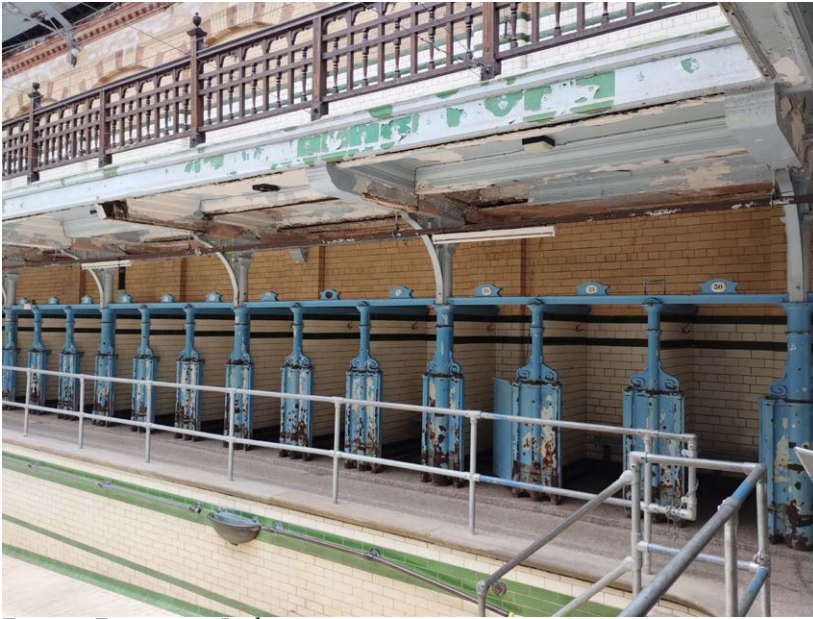
Existing Emergency Lighting
