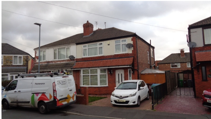
Front Elevation to Application Property.
