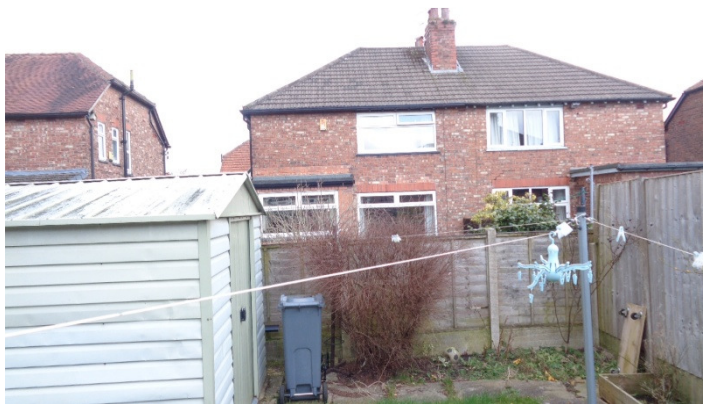
Properties facing Rear Elevation of Application Property.
