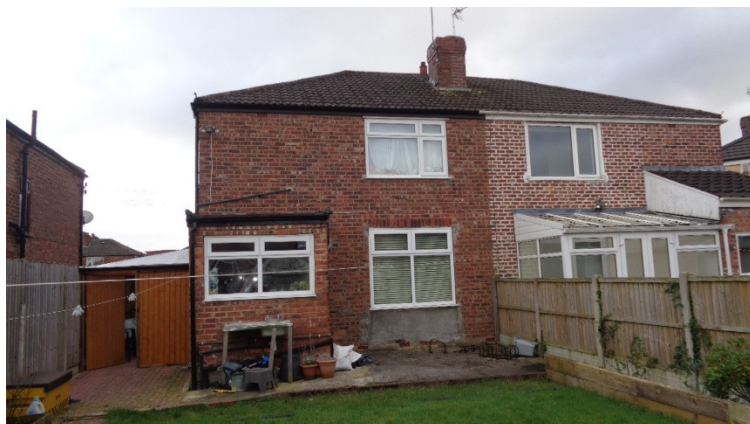
Rear Elevation of Application Property.
