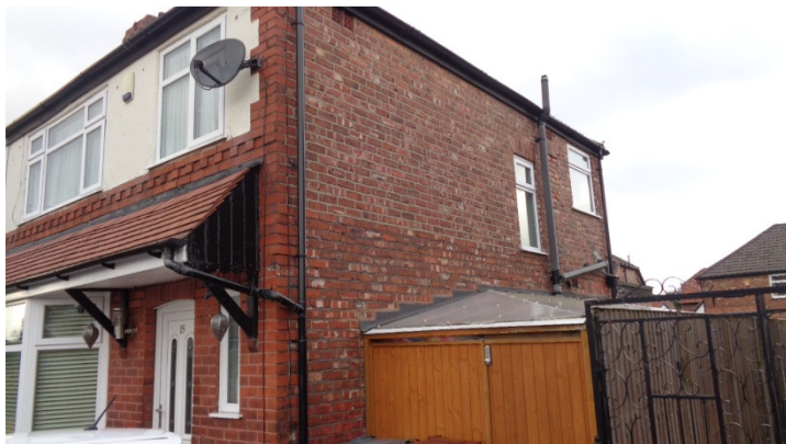
Gable Elevation to Application Property.
