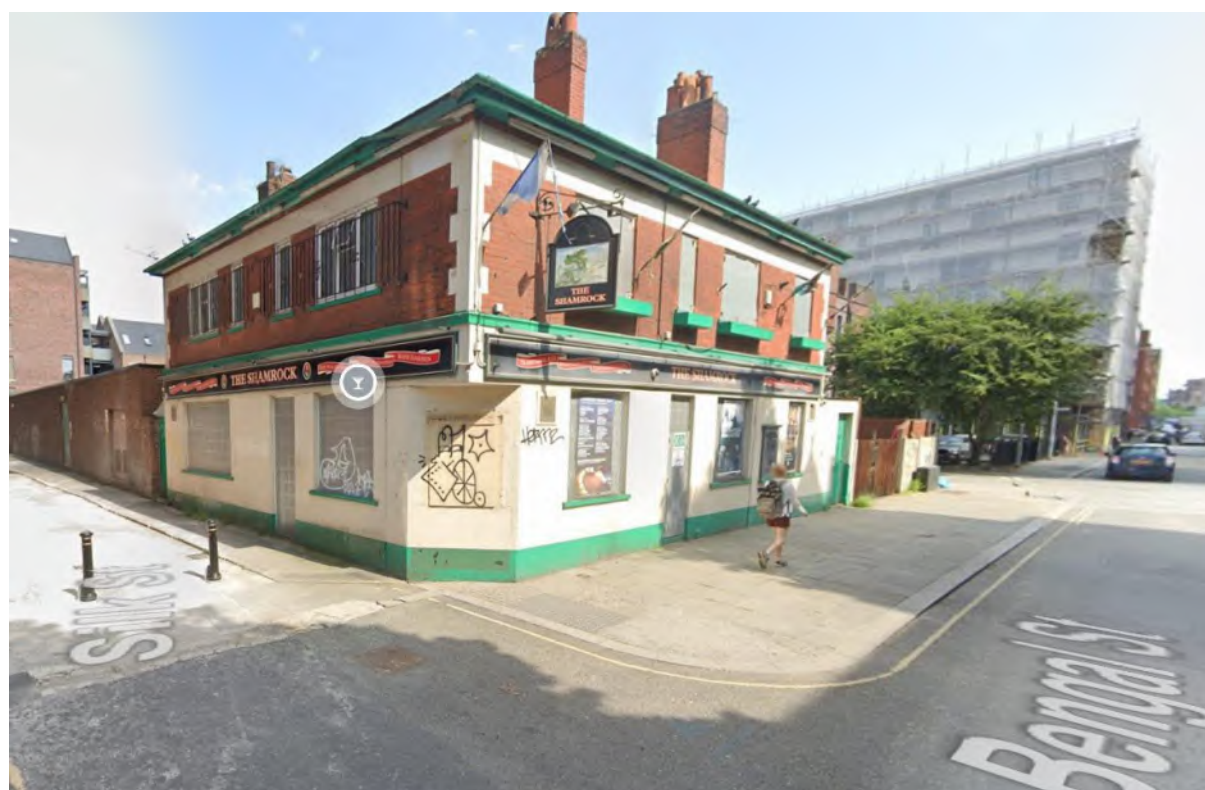
Photo 2 – Looking south at the NW corner of the site
