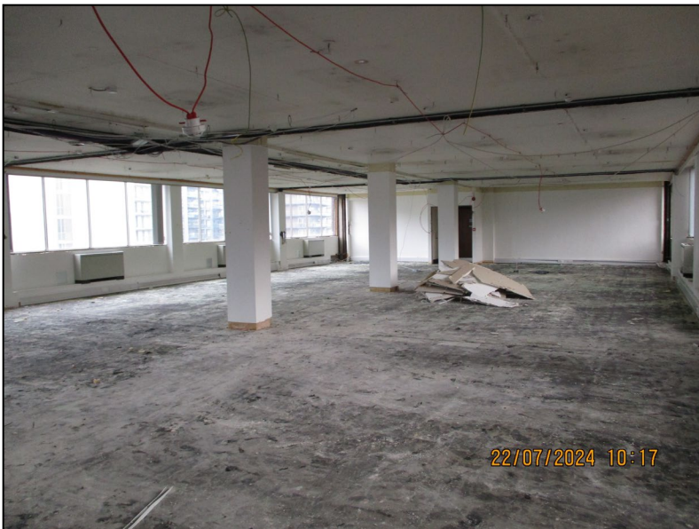
Photo 6 Partially stripped out interior of building
