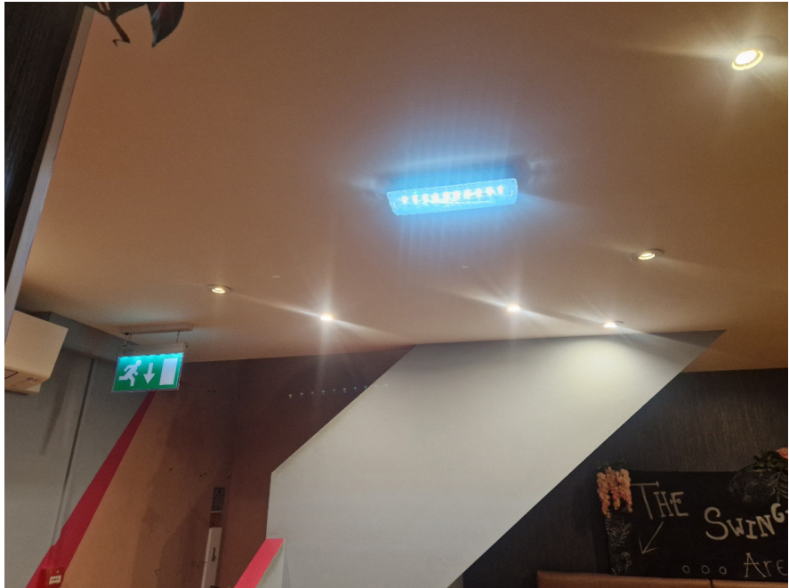
CEILING AND LIGHTING
