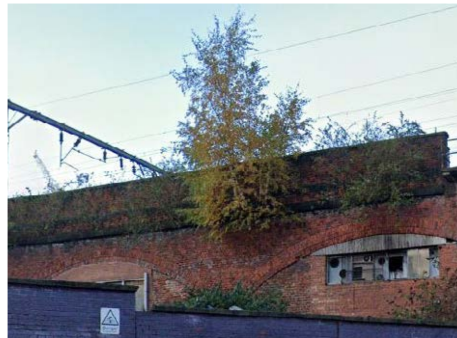
03 Self-seeded Birch tree to existing railway bridge
