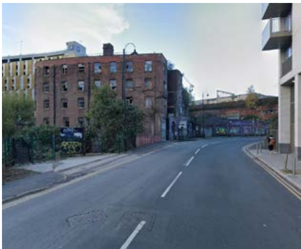
04 View looking north west towards the site on Gloucester Street
