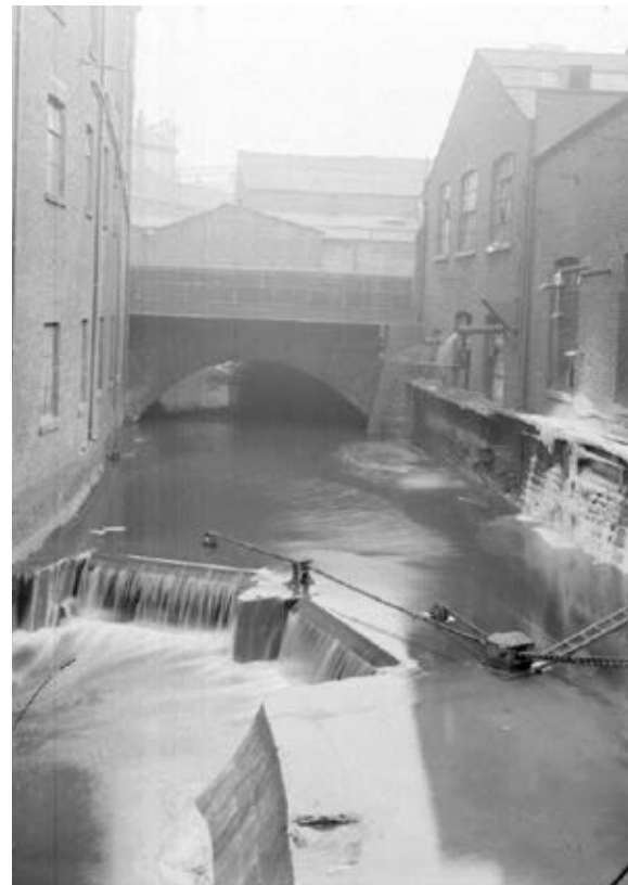
01 Birley's Weir constructed in 1863 to south west corner of the River Medlock
