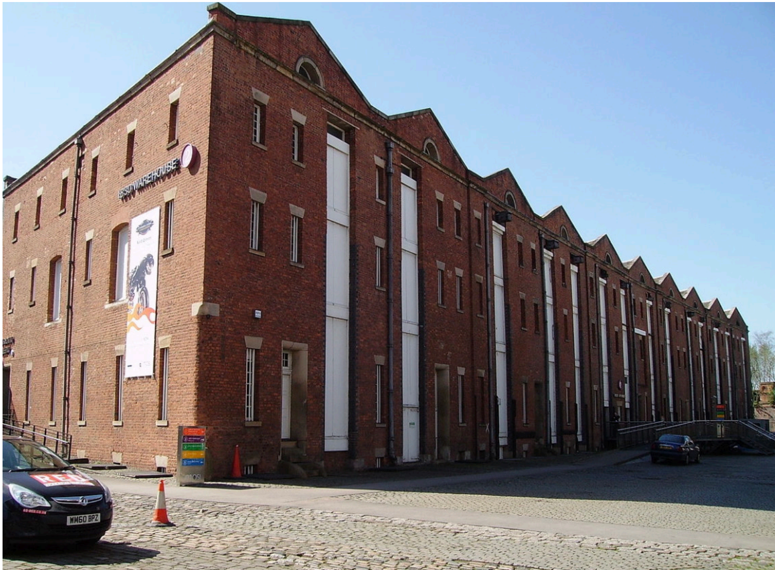
Image: External view of the 1830 Warehouse.
