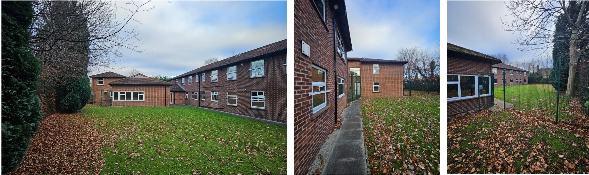
Photographs of the building showing existing building structure, landscaping and security fencing and gates
