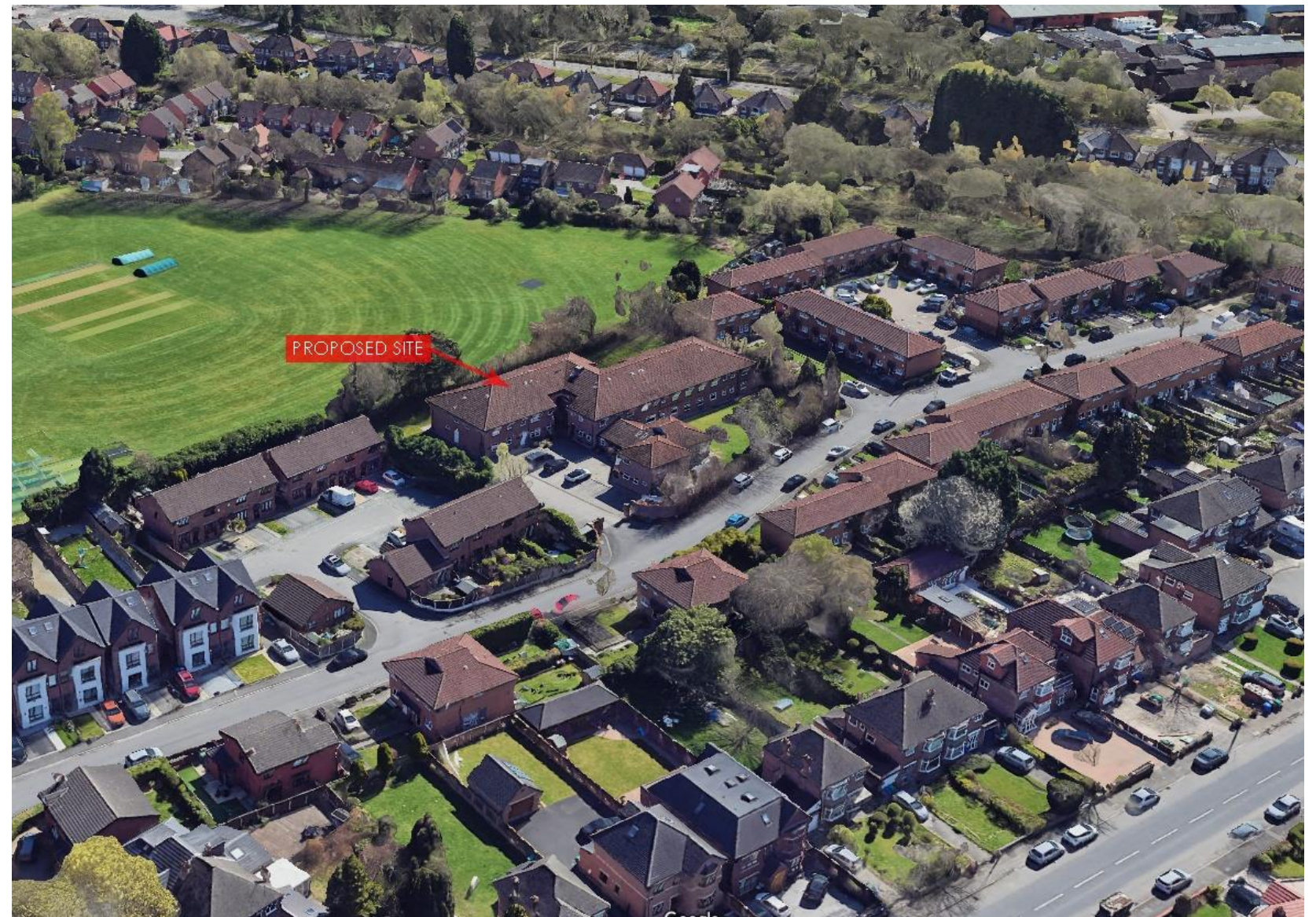
The site location. [Image: Google Maps]
