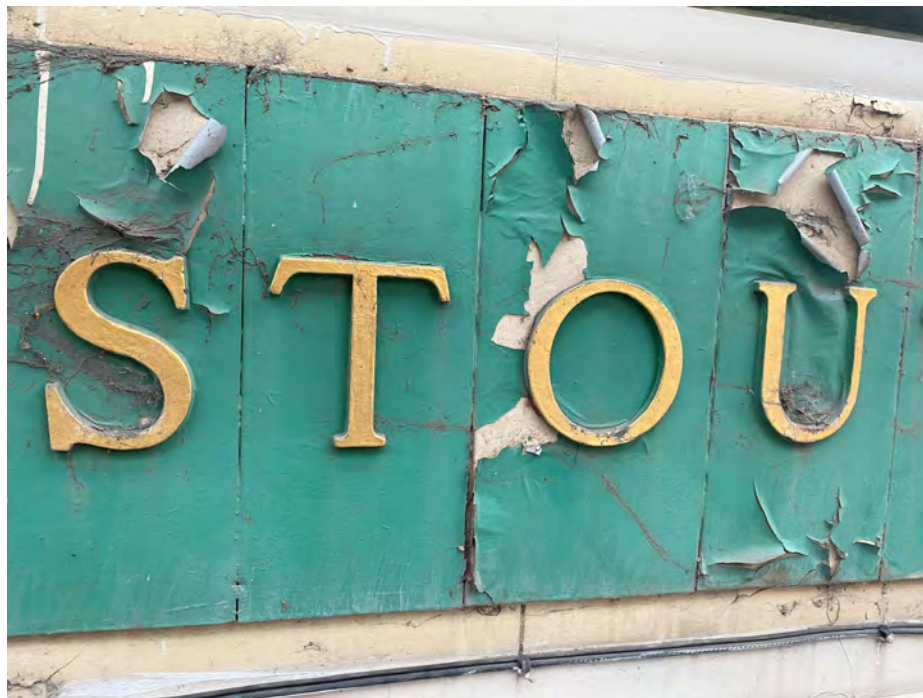
Plate 14 – Relief lettering formed within the individual faience fascia blocks.
