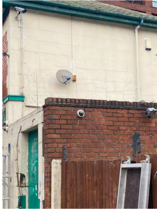
Plate 9 – Lined out render finish to the first floor south elevation.
