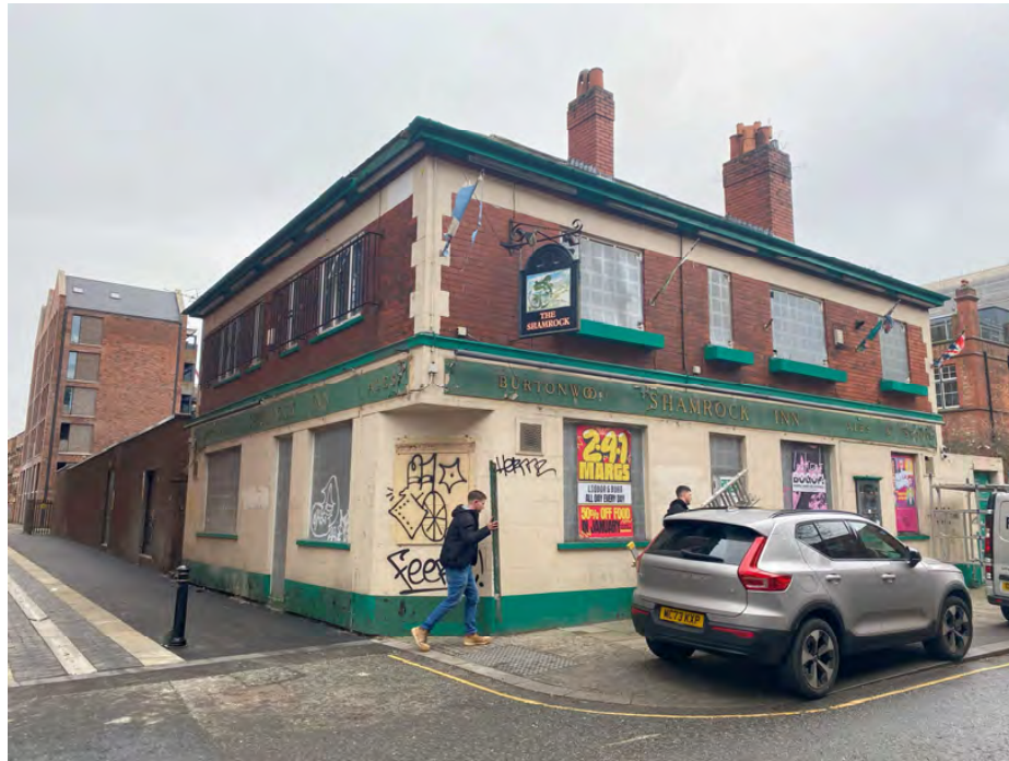
Plate 1 - North and west elevations (following removal of fascia sign board).
