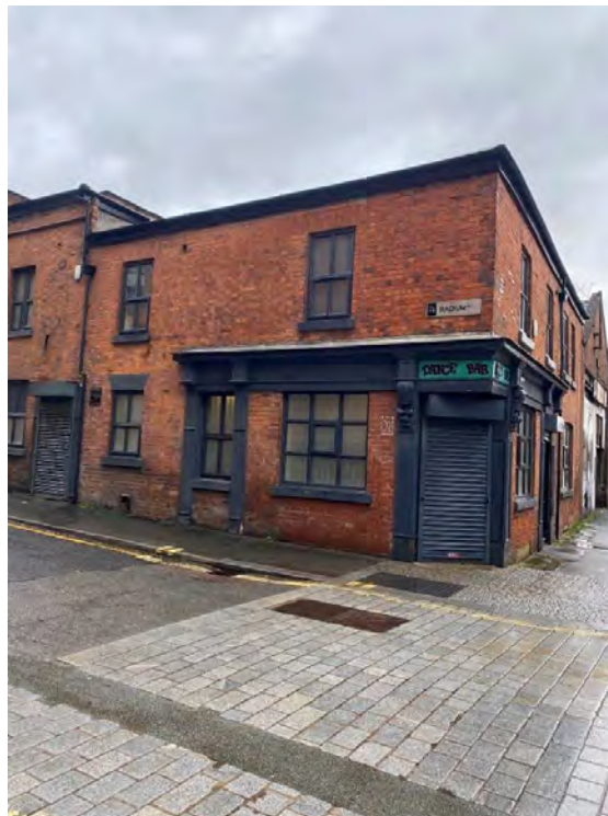
Plate 16 – Former pub to Raglan Street with similar corner feature as The Shamrock.
