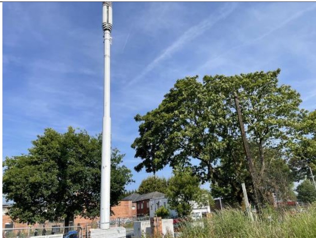
PLATE 8 TELECOMMUNICATIONS MAST ADJACENT TO WESTERN BOUNDARY
