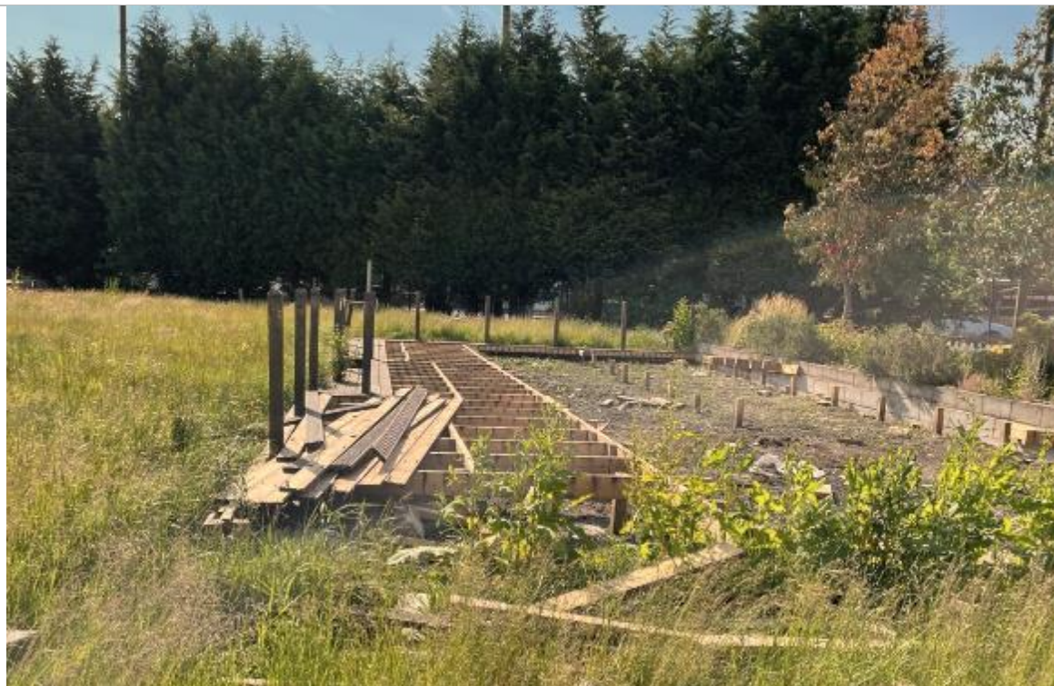
PLATE 7 PARTIALLY DISMANTLED DECKING AND CONFIERS IN SOUTH WEST
