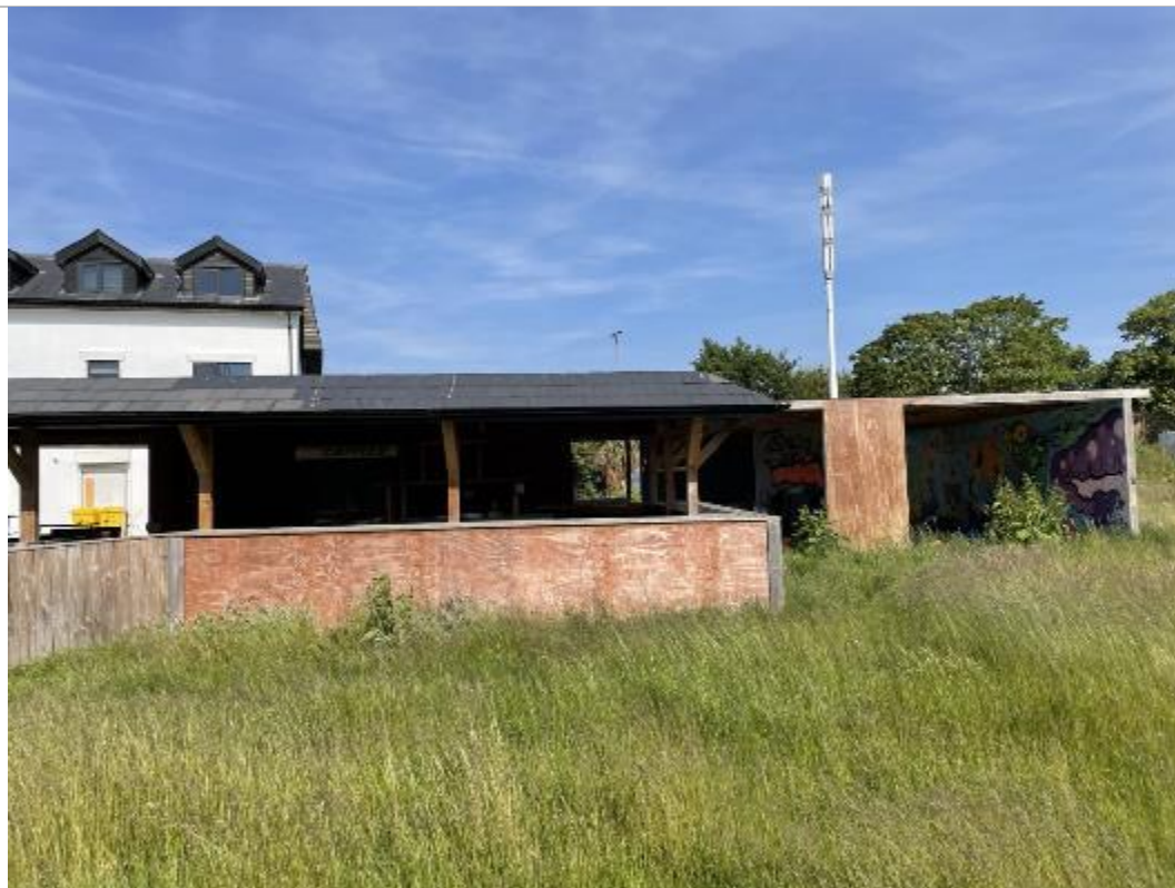
PLATE 7 TIMBER STRUCTURE AT CENTRAL WEST OF SITE
