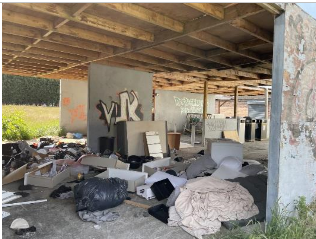
PLATE 5 TIMBER STRUCTURE AND DOMESTIC WASTE IN CENTRAL WEST
