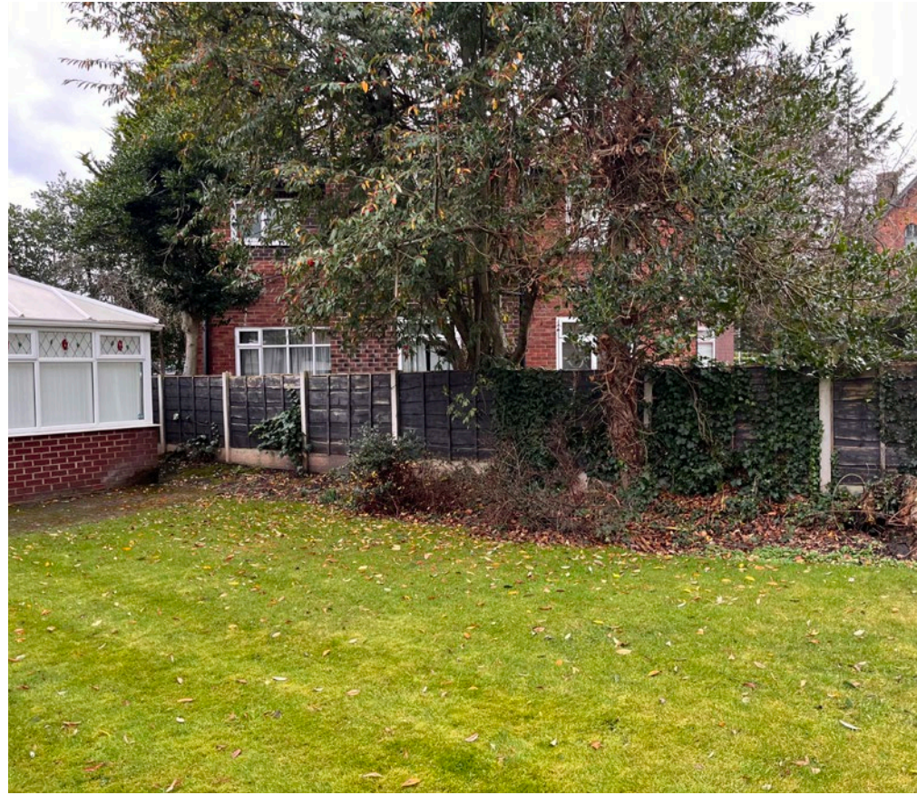
Discuss with the neighbour changing the fence panels
