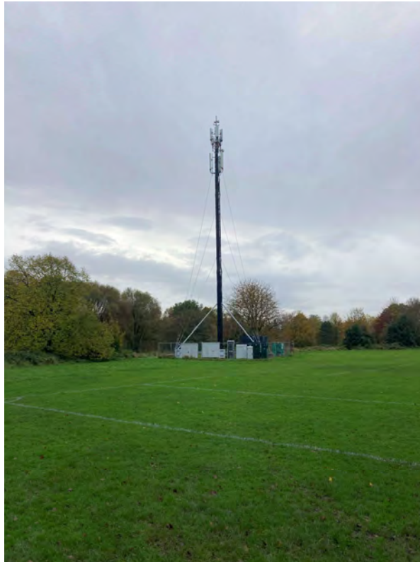
Photo 1: View of the Telecoms Mast
